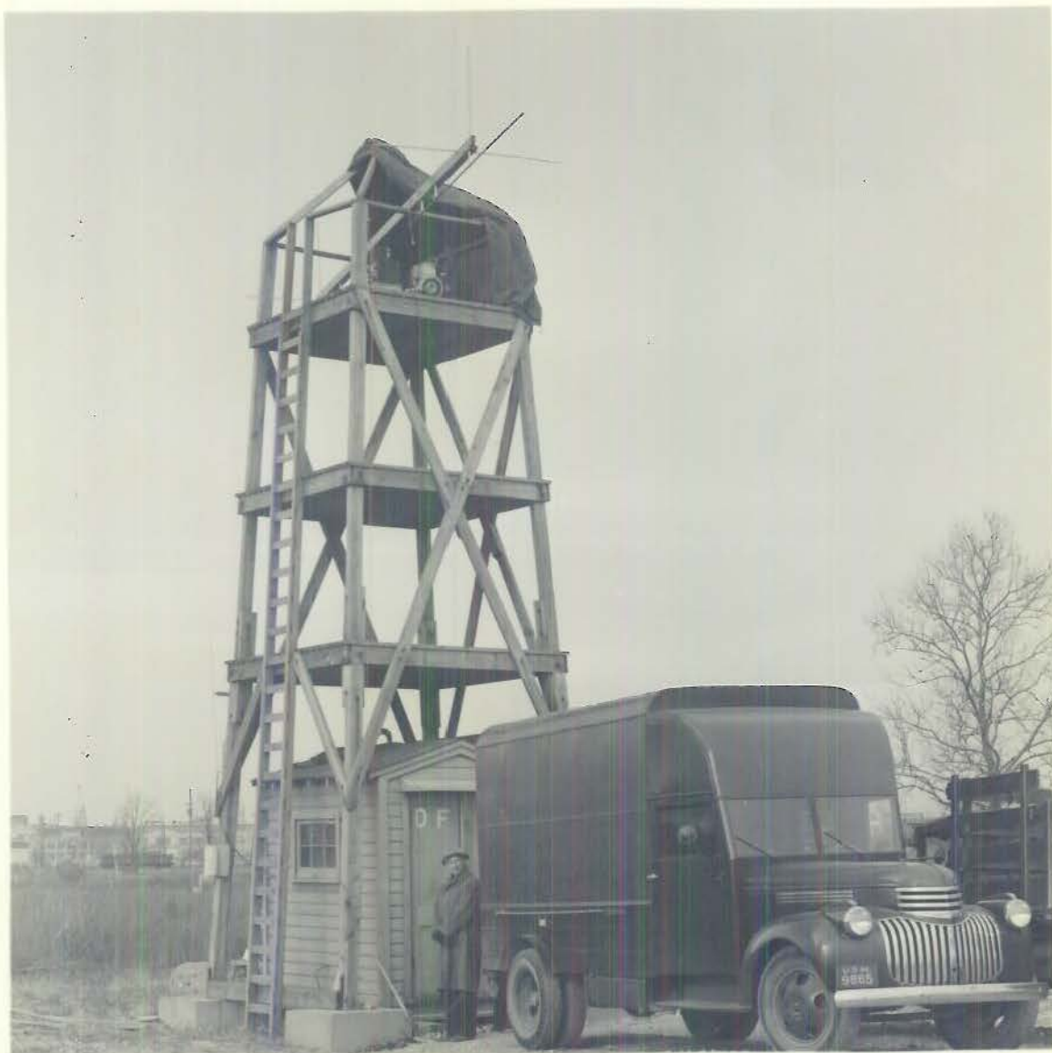
TCS-5 TRANSMITTER (SHOWING GASOLINE POWER GENERATOR)
