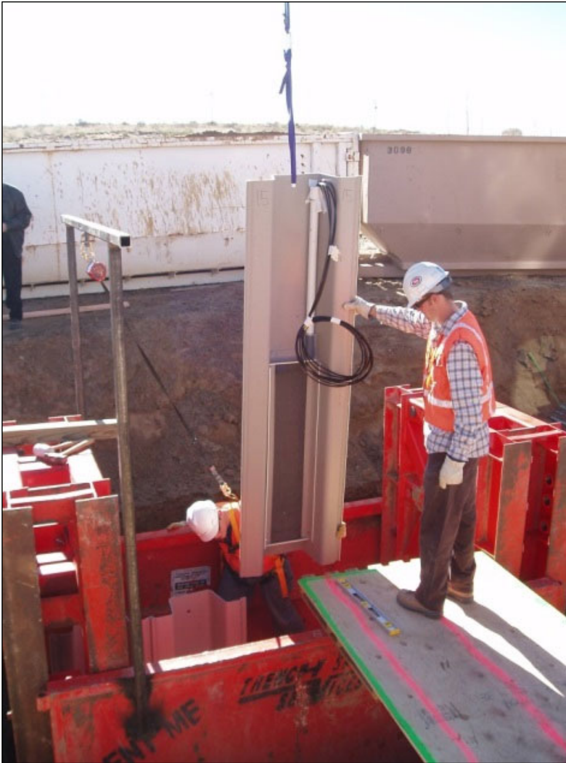
Figure 2: Installation of in situ eBarrier at Pueblo Chemical Depot.
