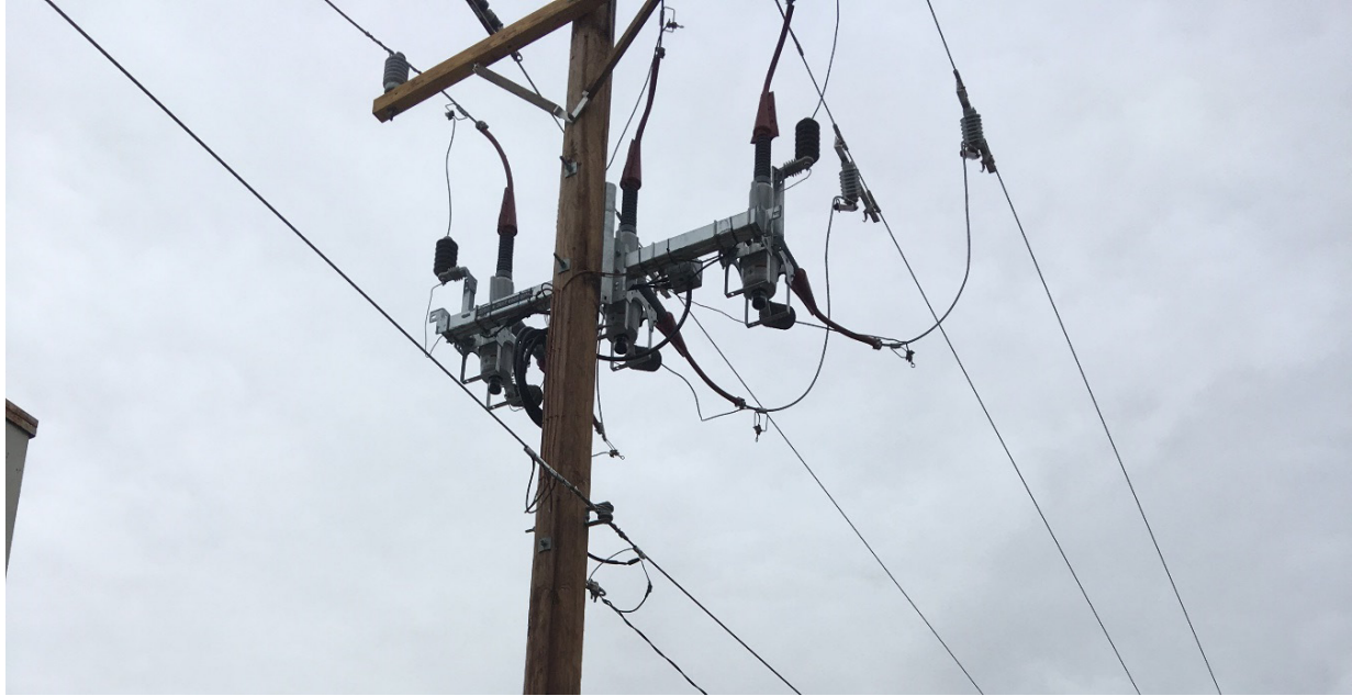
Figure 9. Overhead Recloser
