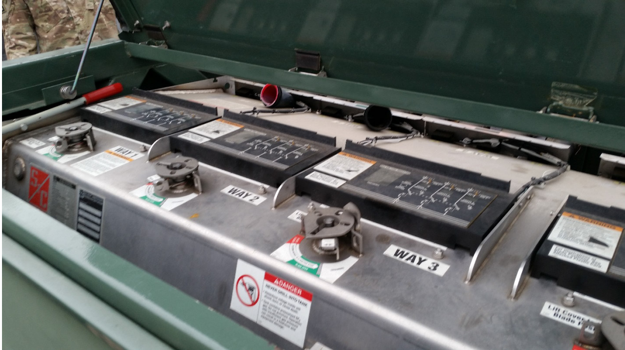
Figure 8. Example S&C Vista Switchgear
