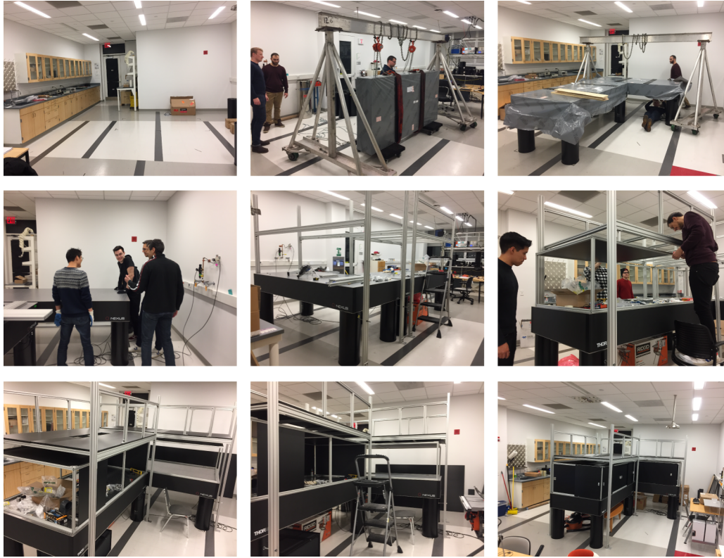
Figure 1: Prior to installing the requested items, we erected the physical infrastructure required to operate the instruments in the form of two optical tables and accompanying canopies and light enclosure boxes. The photo series summarizes our work, starting from an empty room (upper left) to the completed system (lower right).
