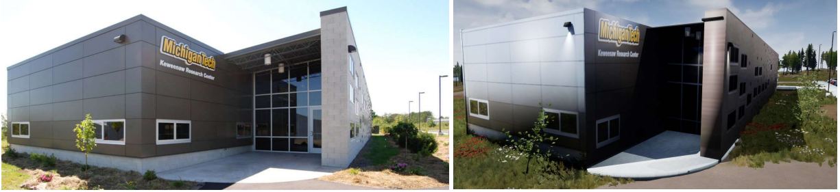
Figure 41 Image (left) and VR visualization (right) of the left side view of the KRC main building.
