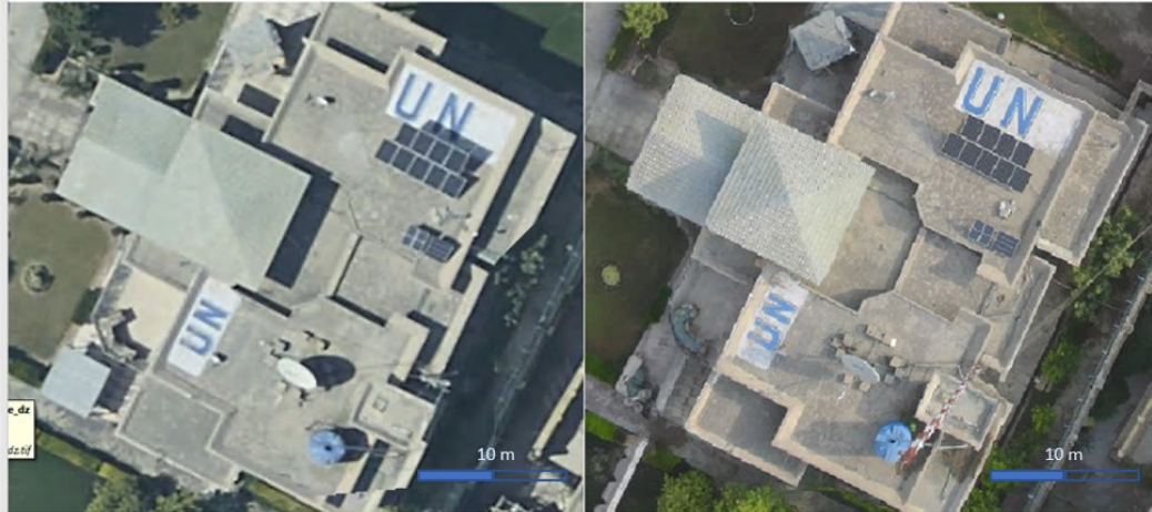
Figure 15. Visual comparison between BuckEye foundation imagery (left) and an individual ARTEMIS/eBee (right) image over a single building in Jalalabad, Afghanistan. The individual shingles and roof texture is visible within the higher spatial resolution ARTEMIS data on the right side.
