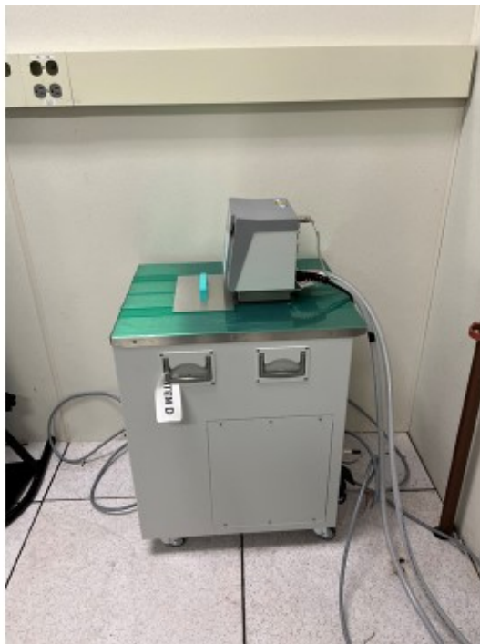
Figure 4. The chiller of the PlasmaPro 100 Cobra ICP etching system in the clean room.
