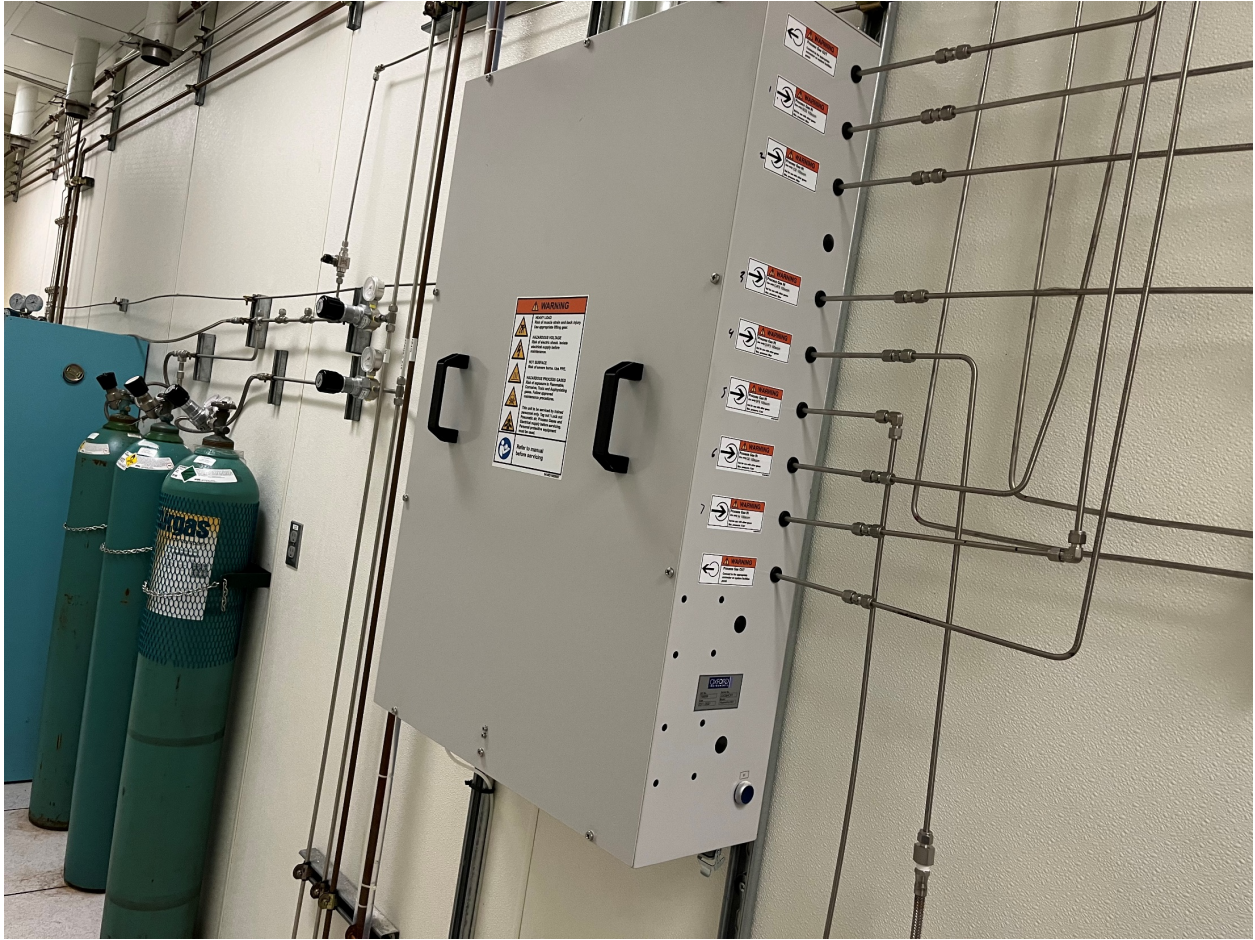
Figure 3. The installed process gas box of the PlasmaPro 100 Cobra ICP etching system in the clean room, which are connected with seven etching process gases including argon (Ar), oxygen (O 2 ), chlorine (Cl 2 ), sulfur hexafluoride (SF 6 ), octafluorocyclobutane (C 4 F 8 ), boron trichloride (BCl 3 ), and Trifluoromethane (CHF 3 ).
