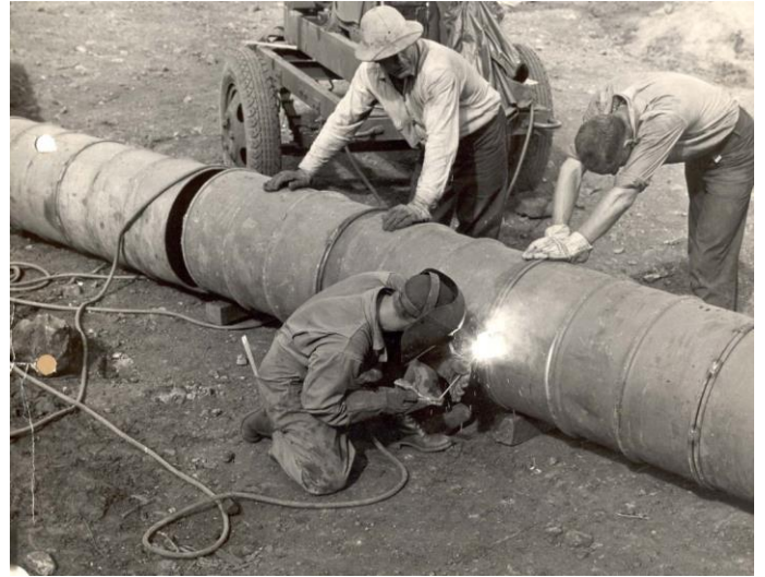
Seabees from the 75th Construction Battalion constructing a sewage pipeline from gasoline
