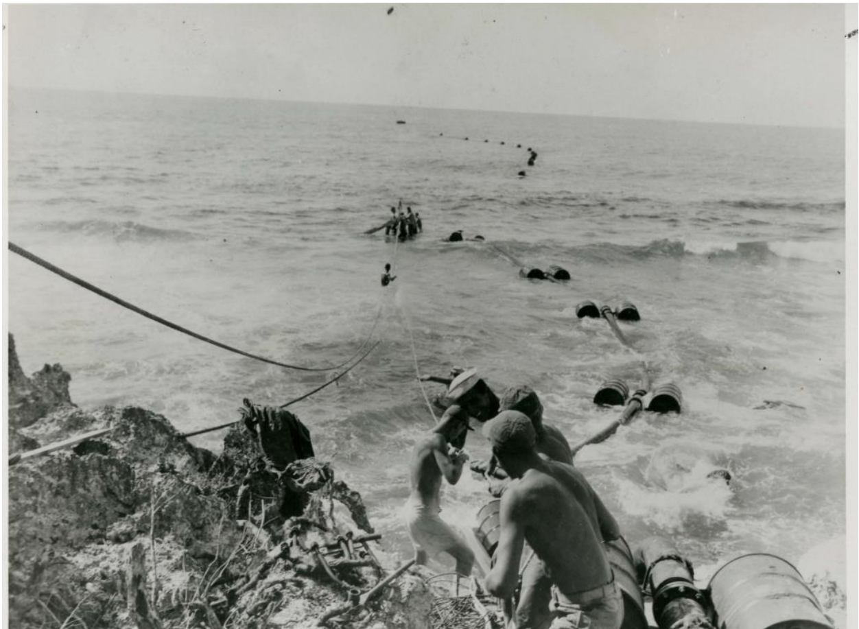
Seabees install submarine pipeline off White Beach, Tinian. They used 55-gallon drums to float the pipeline out to a floating gas station where Submarines could fill up.
