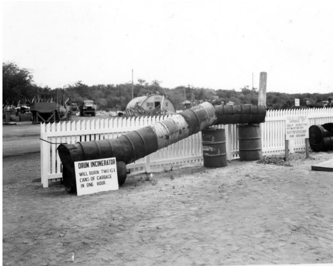
Garbage incinerator made from 55-gallon drums on Okinawa by Seabees with the 81st NCB.
