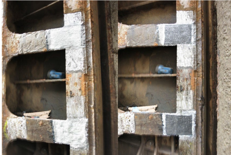
Figure 14. Repairs at locations 1 and 2. At left, glass fiber. At right, carbon fiber.
