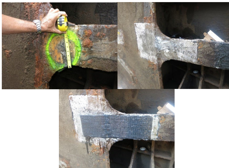
Figure 17. Crack repaired with CFRP at location 6.
