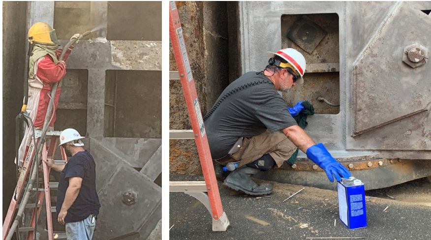
Figure 8. Sandblasting and cleaning the surface with acetone.
