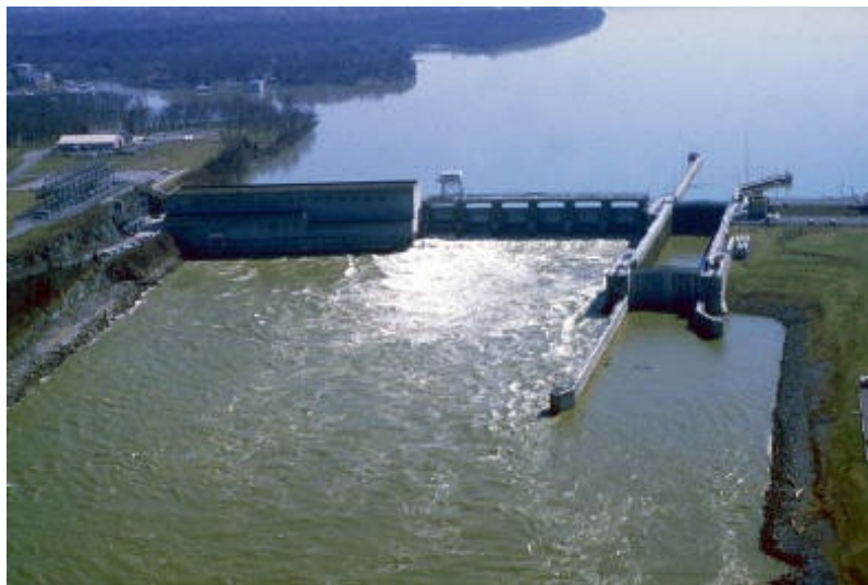
Figure 1. Old Hickory Lock and Dam.
