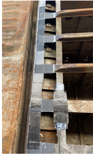
Figure 12. CFRP installation.
