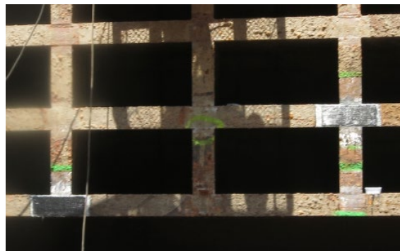
Figure 19. River side showing CFRP repairs when no cracks are present, locations 2 and 3.
