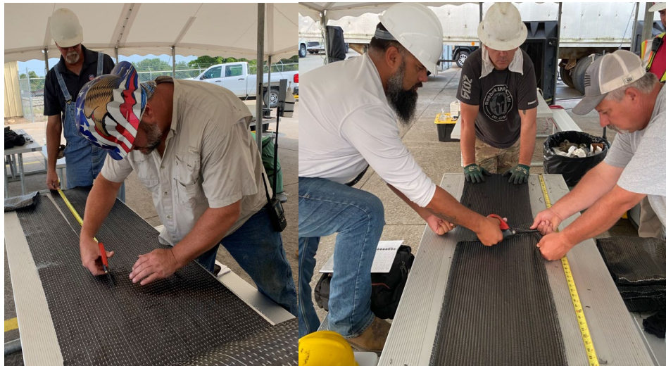
Figure 7. Cutting fibers to specific lengths. At left, CFRP. At right, basalt fibers.
