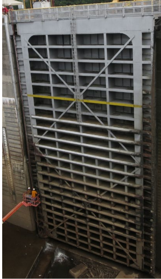
Figure 2. Old Hickory downstream miter gate.
