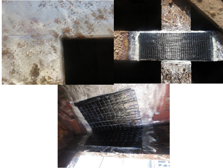
Figure 18. River-side crack repaired with CFRP, location 1.
