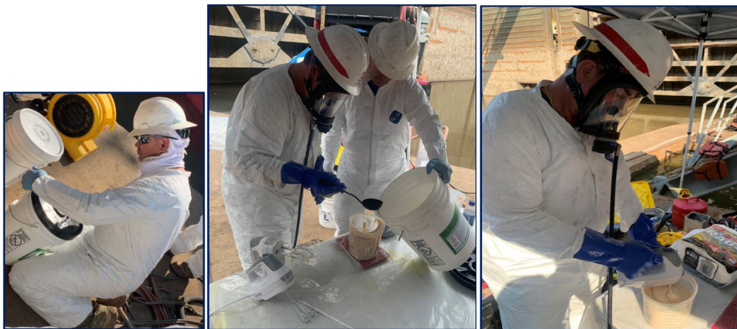
Figure 9. Mixing epoxy and adhesive.
