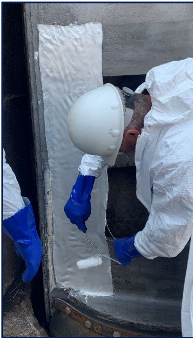
Figure 11. Glass fiber installation.
