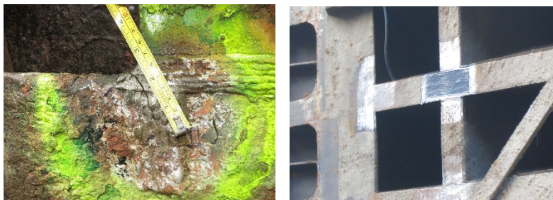
Figure 20. River-side crack repaired with CFRP.
