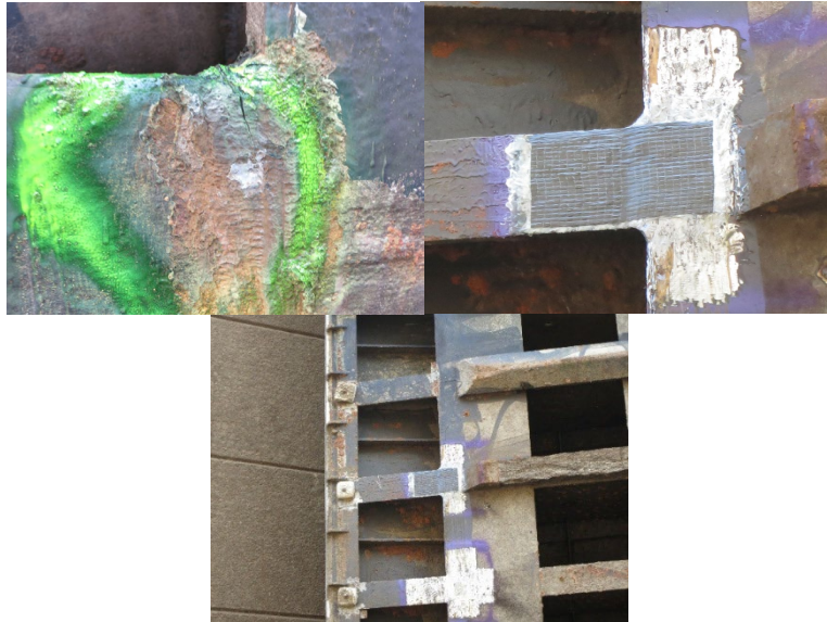
Figure 16. Welded crack repaired with CFRP at location 5.
