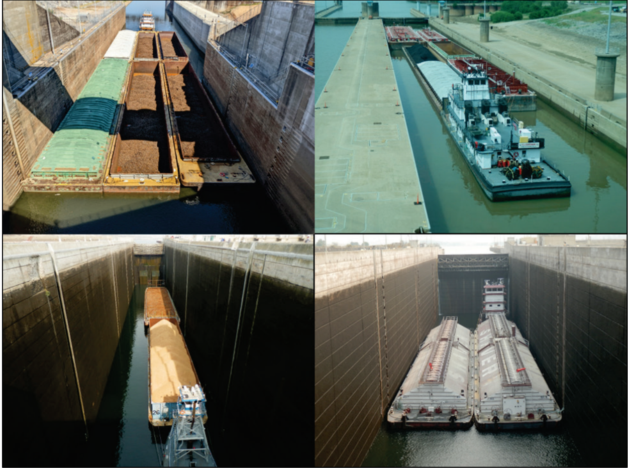
Figure 4. Various barge tow configurations at USACE locks.
