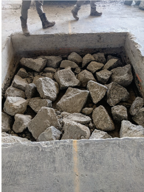
(a) Placement of 12 in. debris
