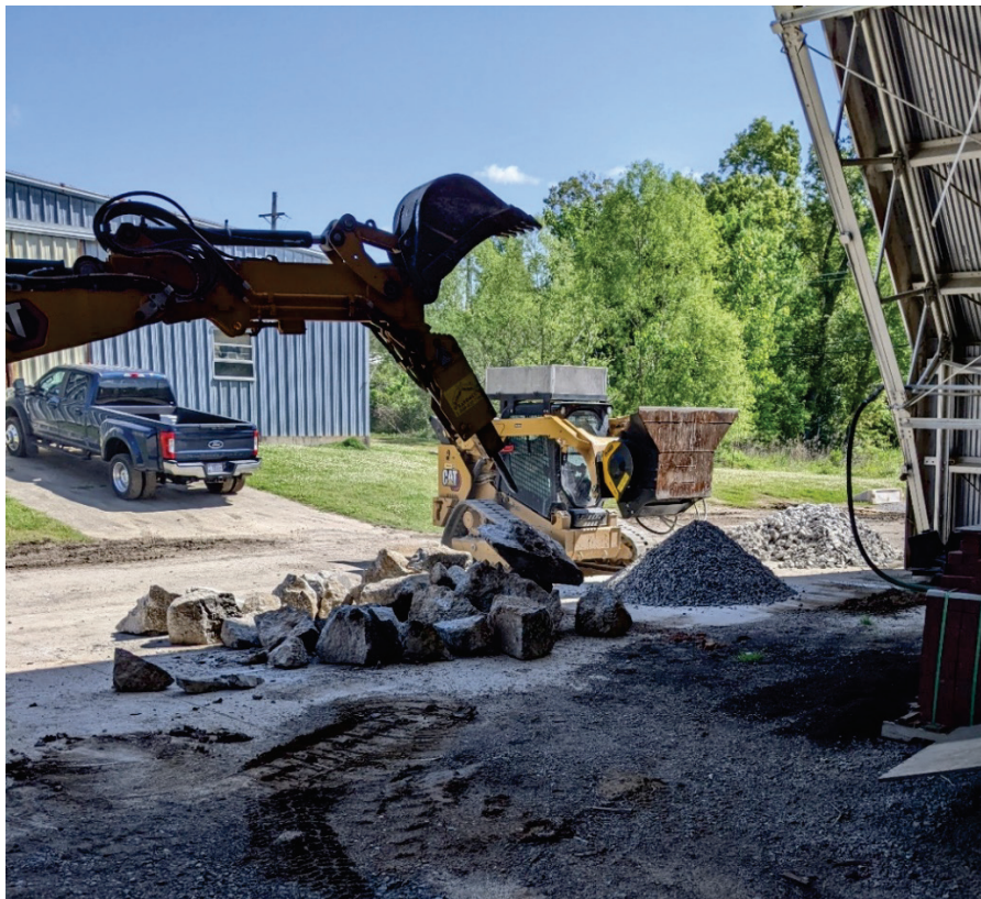
Figure 100. Processing debris backfill.
