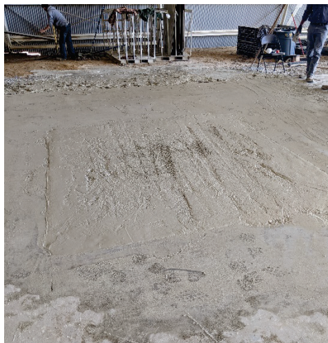
(f) Completed rapid set crater surface
