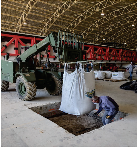
(a) Positioning flowable fill over crater
