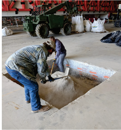
(b) Spreading flowable fill to a uniform thickness
