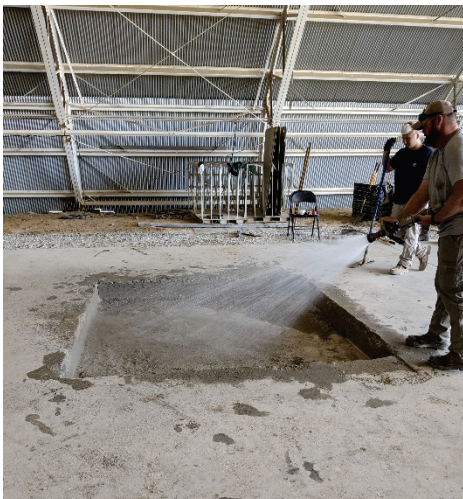
(c) Applying water to flowable fill layer
