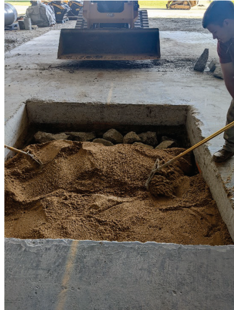
(b) Placement of sand layer over 12 in. debris
