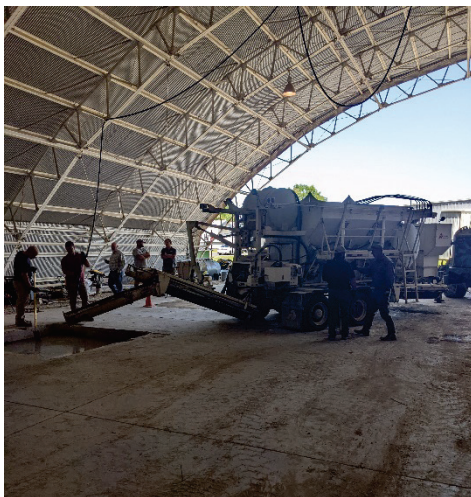
(e) RS mixture placement with volumetric mixer
