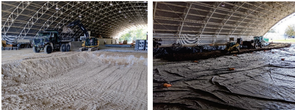
(a) John Deere 130G tracked excavator
