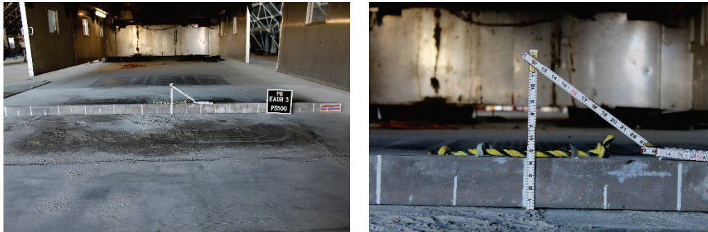
(a) Overall view
