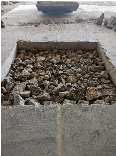
(c) Placement of 9 in. debris
