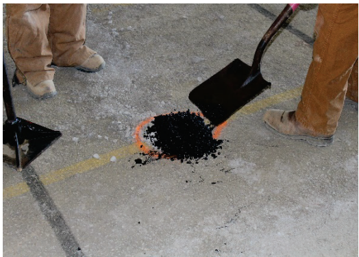
(c) Covering with HMA
