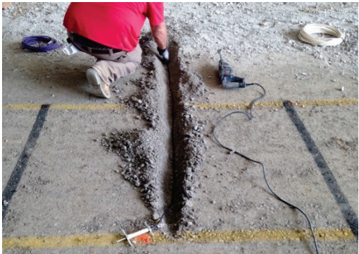
(a) Trenching for wire
