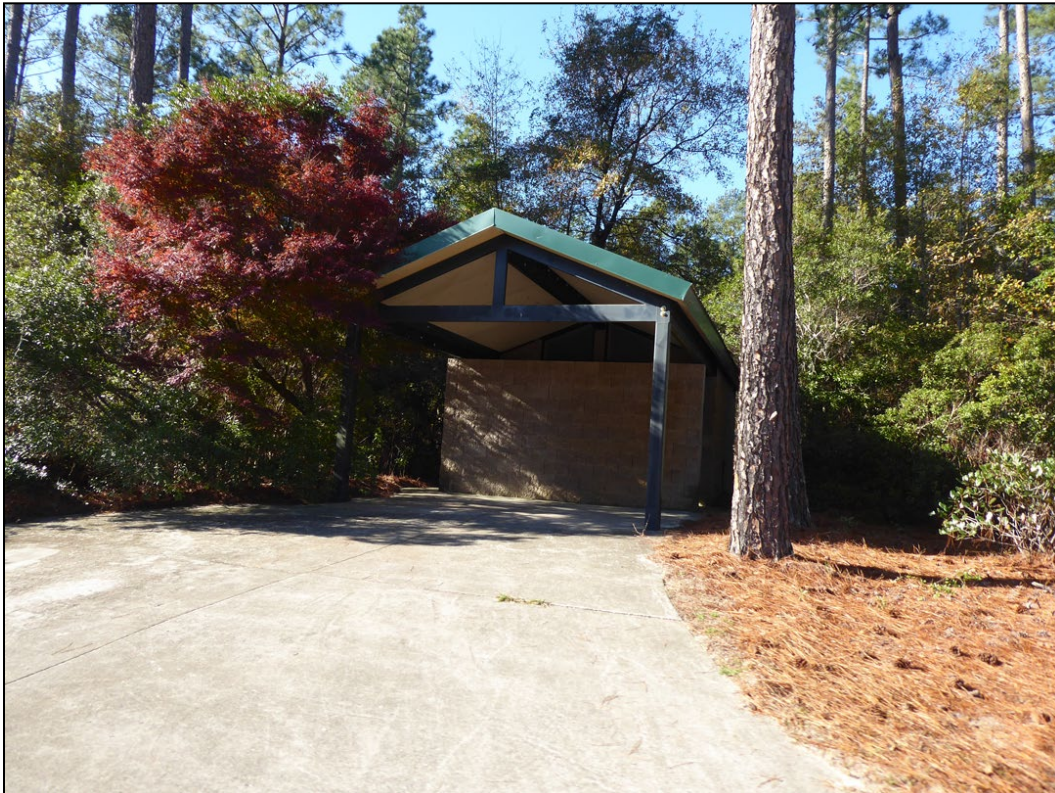
Figure 62. View of Building 545 (Bathroom/Showers), constructed in 2007. (ERDC-CERL, 2020. Public domain.)
