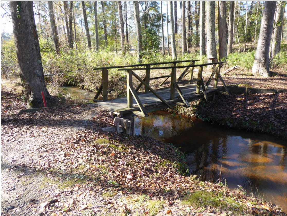
Figure 49. View of GL009 (pedestrian bridge) that dates to 1976. (ERDC-CERL, 2020. Public domain.)
