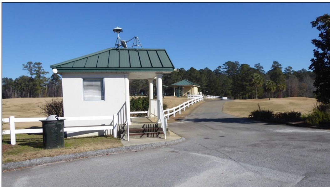
Figure 38. Looking northeast along the path on the southeast side of GL019 (Driving Range) with Building 536 in the foreground and Building 541 in the distance. (ERDC-CERL, 2020. Public domain.)
