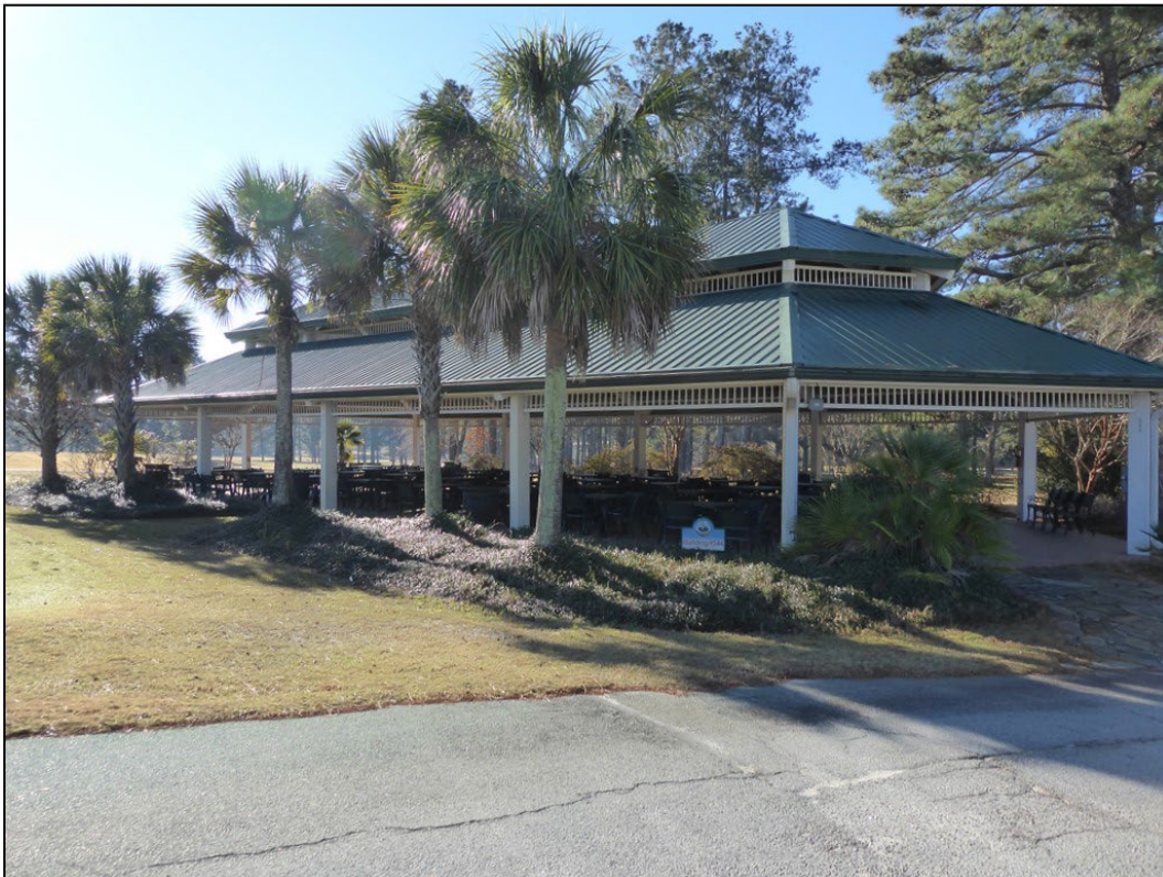
Figure 61. Looking south at Building 544 (Pavilion). (ERDC-CERL, 2020. Public domain.)
