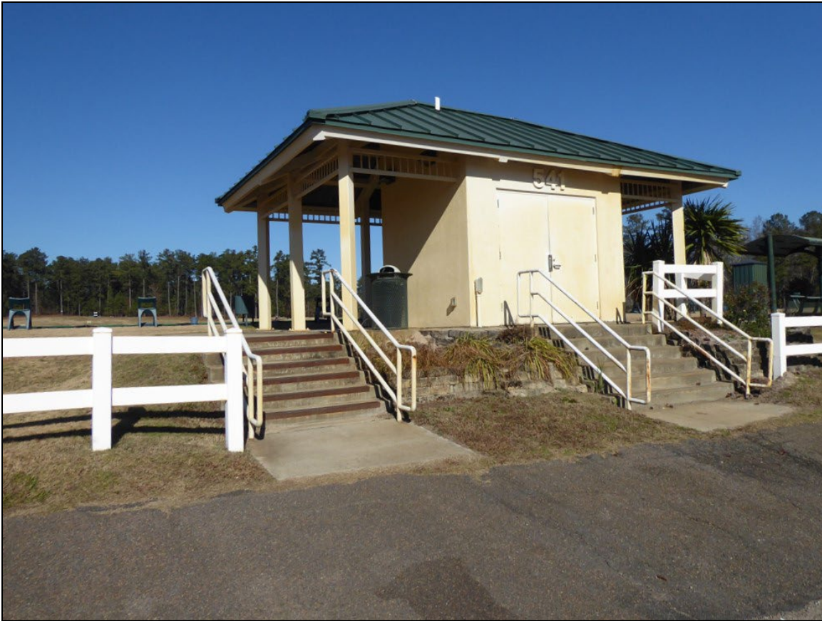
Figure 59. Looking northwest at Building 541 (Range Ball Facility). (ERDC-CERL, 2020. Public domain.)
