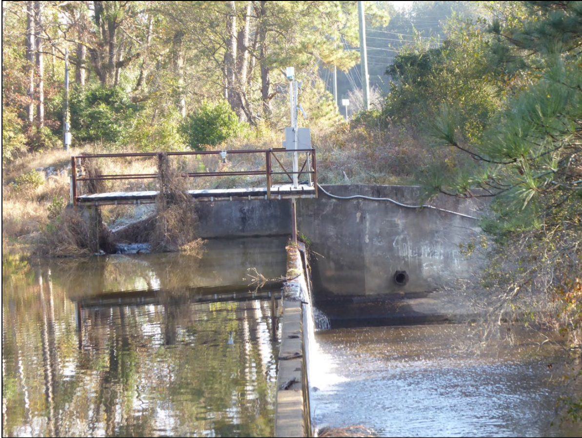
Figure 16. Looking north at Gordon Lake dam. (ERDC-CERL, 2020. Public domain.)
