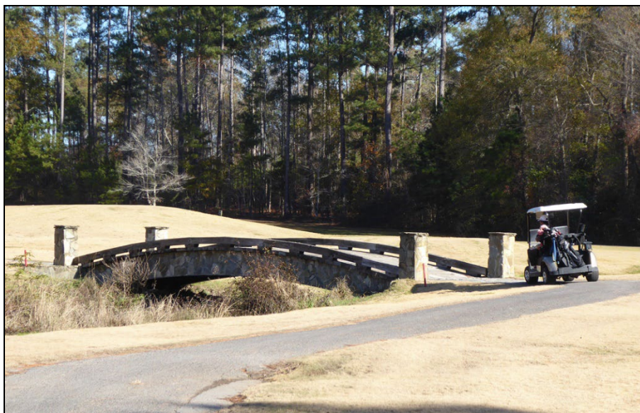
Figure 63. View of ISLD7, which is a glue lam and timber decked bridge erected in 2009. (ERDC-CERL, 2020. Public domain.)
