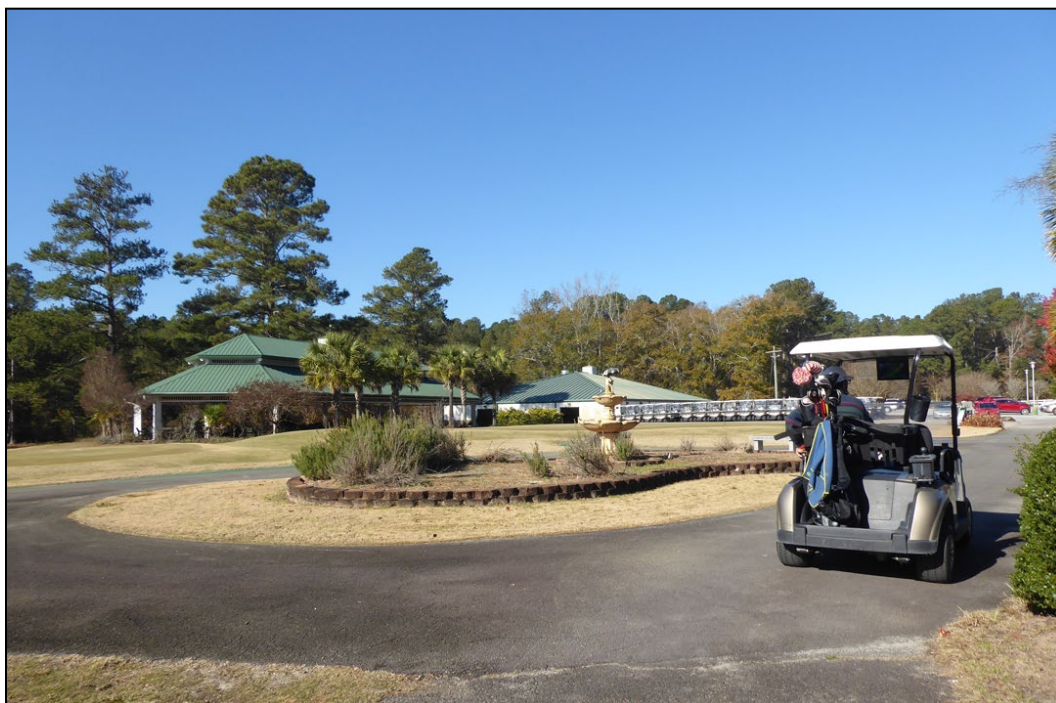
Figure 20. Pavilion, constructed 2007, at Gordon Lakes Golf Club. (ERDC-CERL, 2020. Public domain.)
