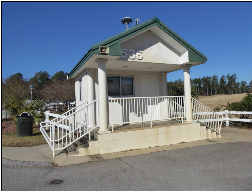
Figure 19. Recreation support building/shed/starter shack, constructed in 2009, at Gordon Lakes Golf Club. (ERDC-CERL, 2020. Public domain.)
