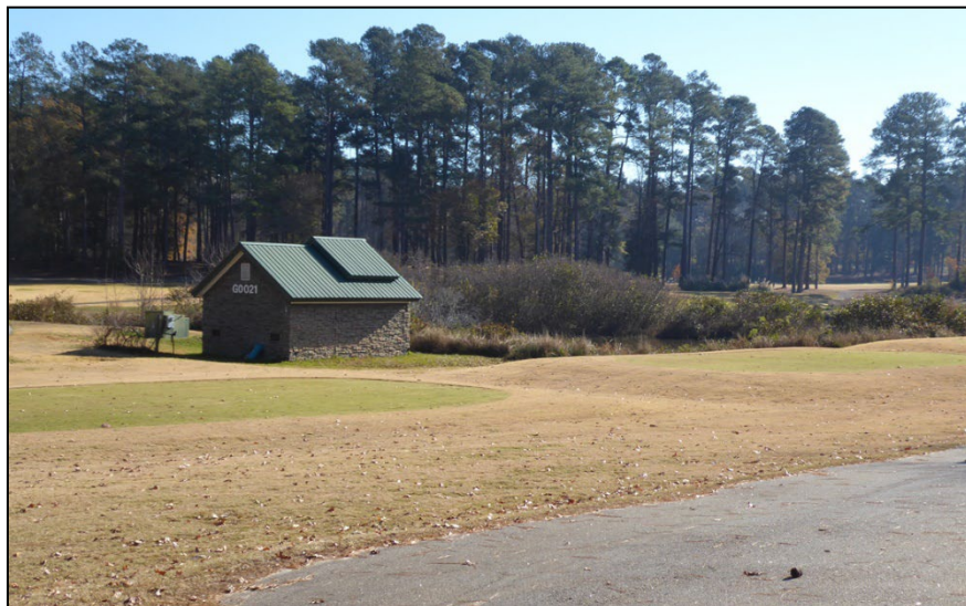
Figure 44. View of G0021, which is the water intake building for the golf course, constructed in 2002. (ERDC-CERL, 2020. Public domain.)
