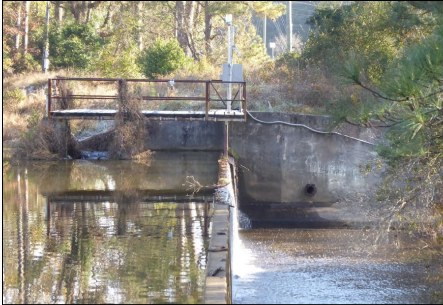
Figure 47. Detail of Gordon Lake Dam. (ERDC-CERL, 2020. Public domain.)
