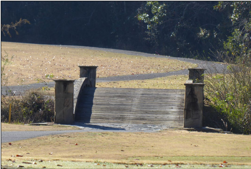
Figure 17. A footbridge at Gordon Lakes Golf Club added to the landscape in 2009. (ERDC-CERL, 2020. Public domain.)
