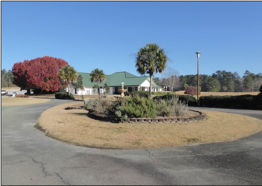
Figure 56. Looking northwest to Building 537 (Clubhouse), constructed in 1975 and modified in the 2000s. (ERDC-CERL, 2020. Public domain.)
