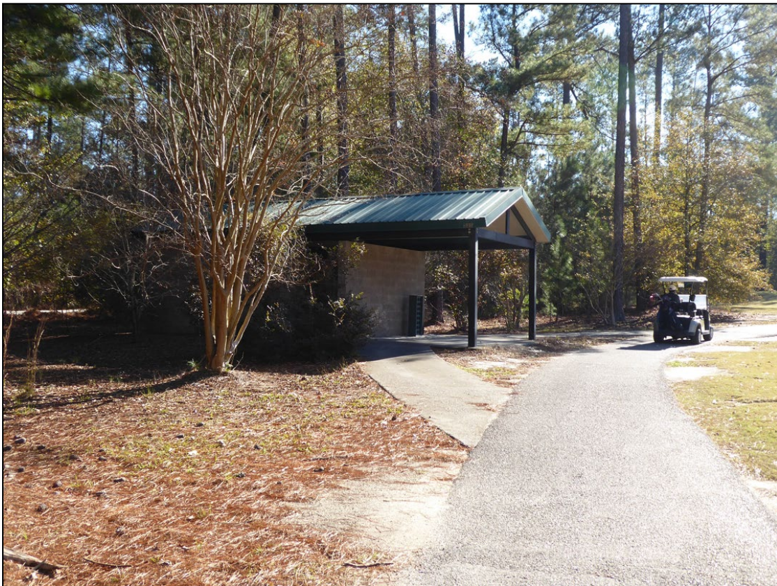
Figure 50. View of Building 535 (Bathroom/Showers), constructed in 2007. (ERDC-CERL, 2020. Public domain.)
