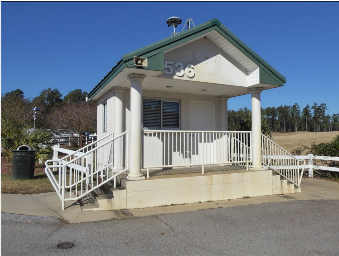
Figure 51. Looking west at Building 536 (REC Support Building), constructed in 2009. (ERDC-CERL, 2020. Public domain.)
