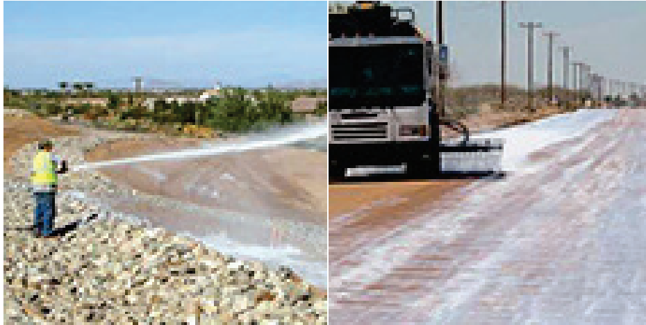
Figure 5. Soiltac application (Soilworks 2020).
