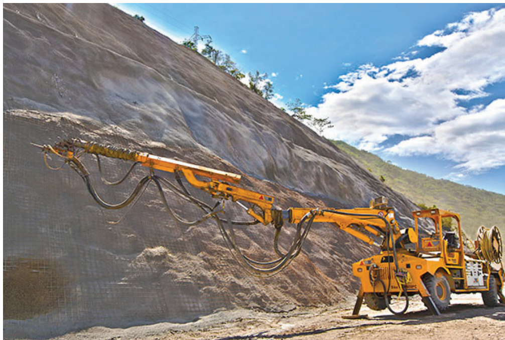
Figure 1. Shotcrete for high-slope, high-height applications (Putzmeister 2019).
