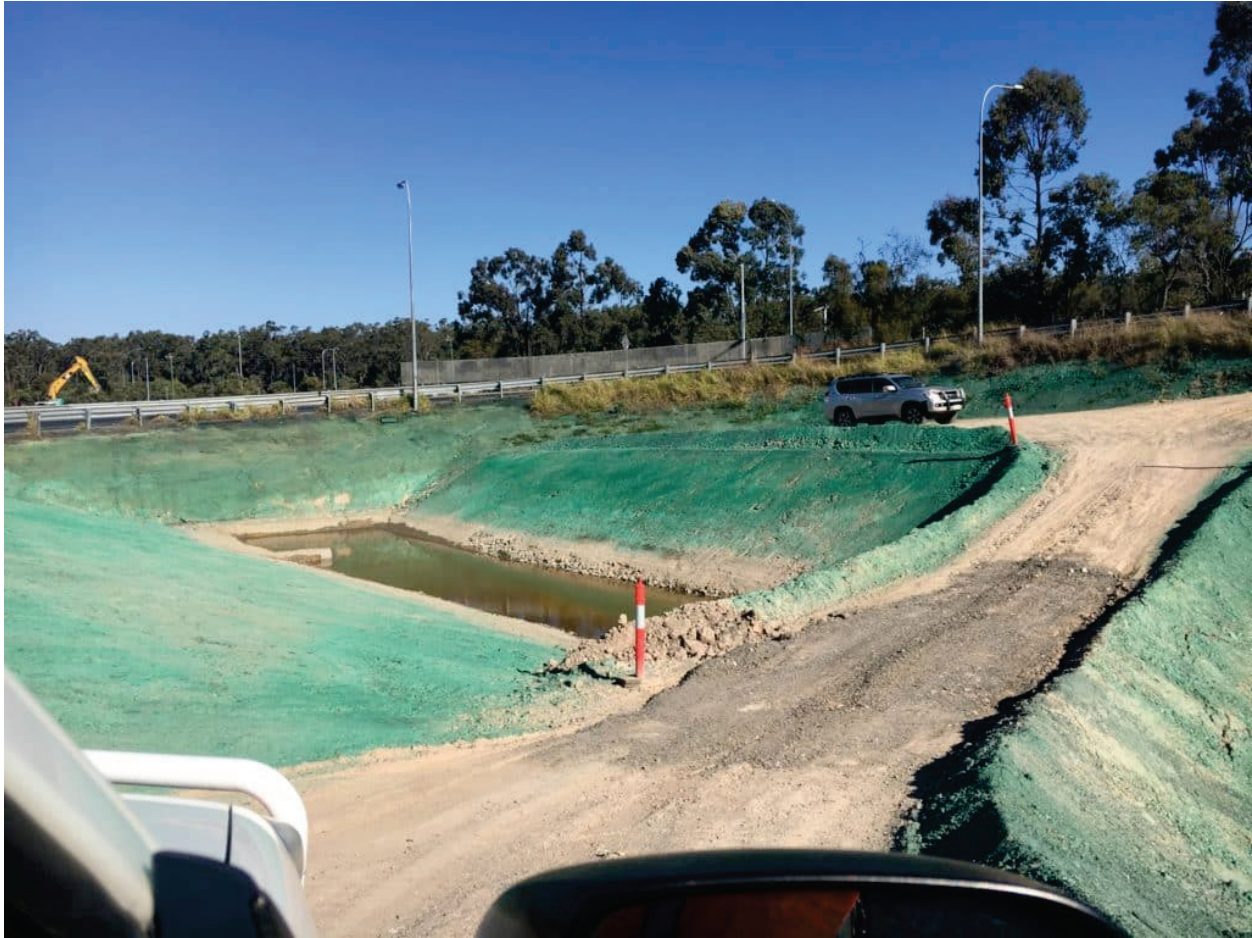
Figure 8. Interchanged embankment (GRT 2019).
