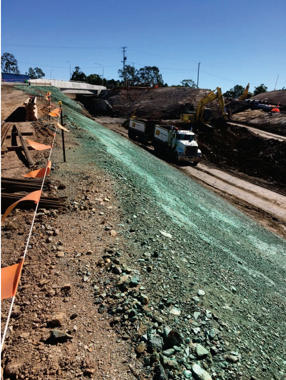
Figure 7. Light rail embankment (GRT 2019).
