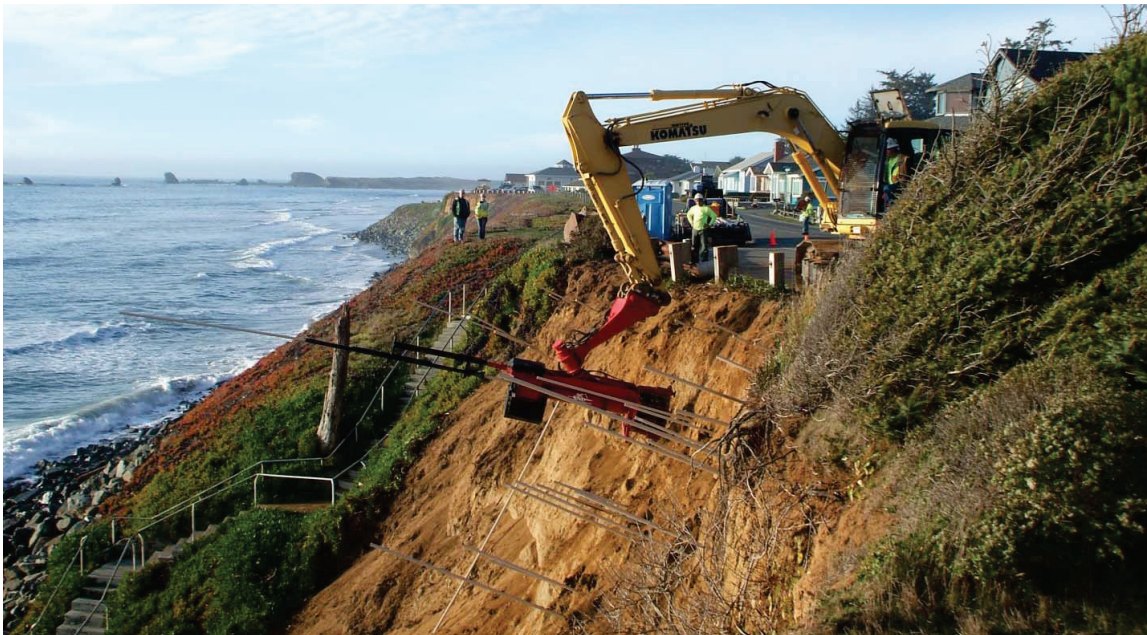
Figure 2. Soil nailing (Chinchiolo and Barret 2011).
