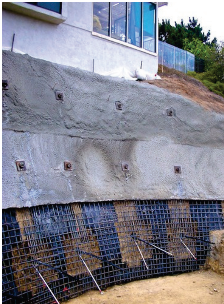
Figure 3. Shotcrete retaining wall (Soil Engineering Construction 2020).
