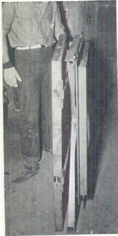
THERMIT MOUNTING FIXTURE FOLDED UP AND READY FOR TRANSPORTATION
