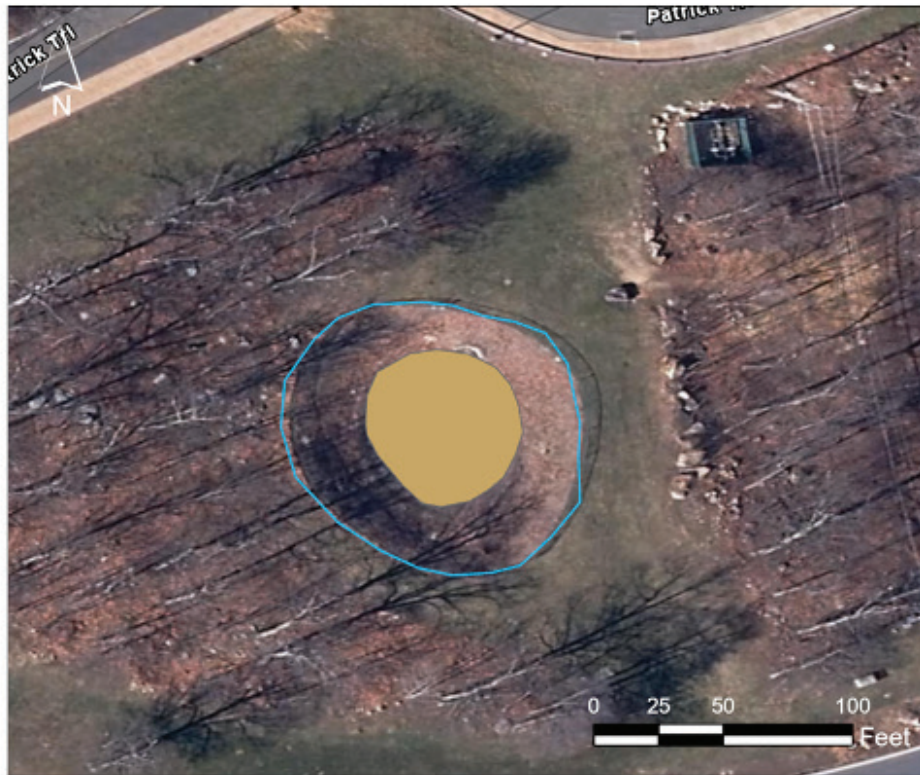
Figure D-8. Detention pond (zoomed in) at Child Development Center at Patrick Trail and Stony Lonesome Rd., US Army Garrisons, West Point, NY.
