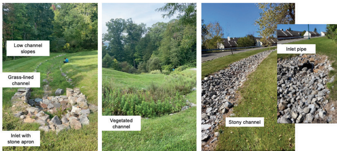
Figure 4. Example of stony and grass swale components at USAG West Point.
