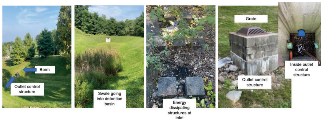
Figure 5. Detention basin components.
