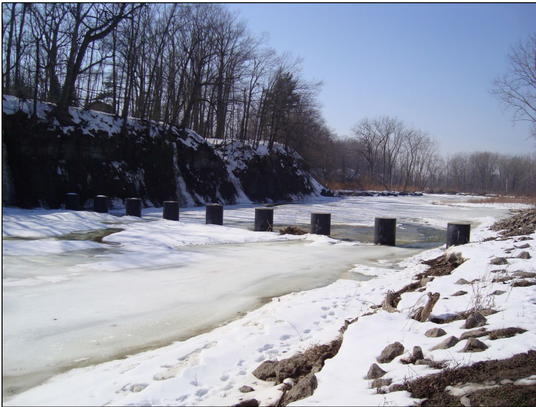
Figure 35. Ice control pier structures, Cazenovia Creek, New York (Image reproduced from USACE Buffalo District. Public domain.)
