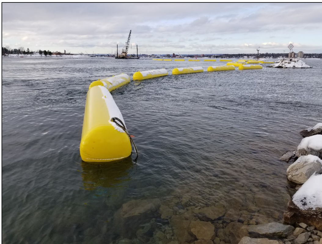
Figure 34. Example of ice boom arrangement, St. Marys River, Michigan. (Image reproduced from USACE Soo Project Office. Public domain.)
