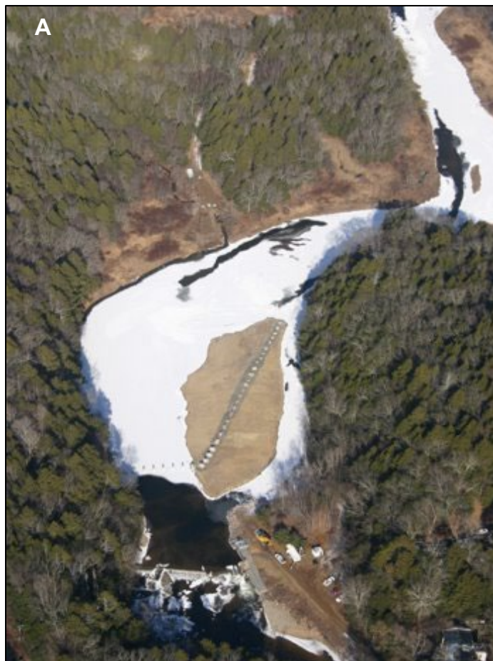
Figure 36. Ice control using concrete pier structures Salmon River, Connecticut. Prior to melt out (A) (Google Earth) and after (B). Note debris buildup upstream of pier structures (B).
