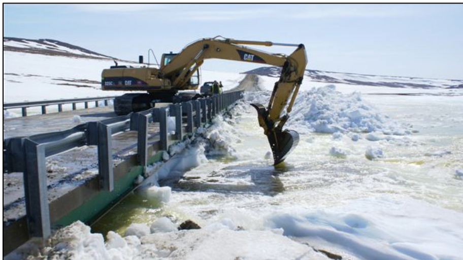
Figure 31. Excavator removing jammed ice from underneath a bridge near Nome, Alaska (Photo: Alaska Department of Transportation, used with permission).
