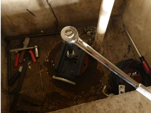
Figure 3. Removing transducer with second version of Transducer puller.
