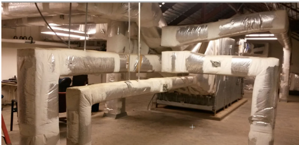
Multizone air handlers mix a zone specific air temperature for each zone, which has its own dedicated duct
