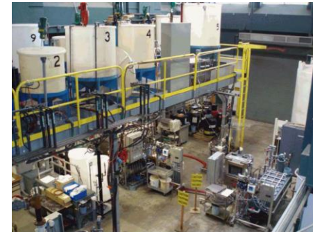
NSWCCD Wastewater Lab
