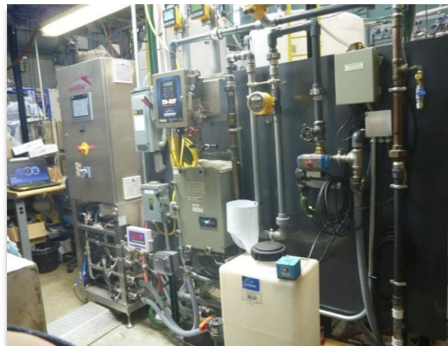
3) Influent processed through system; effluent analyzed by oil content monitors.
