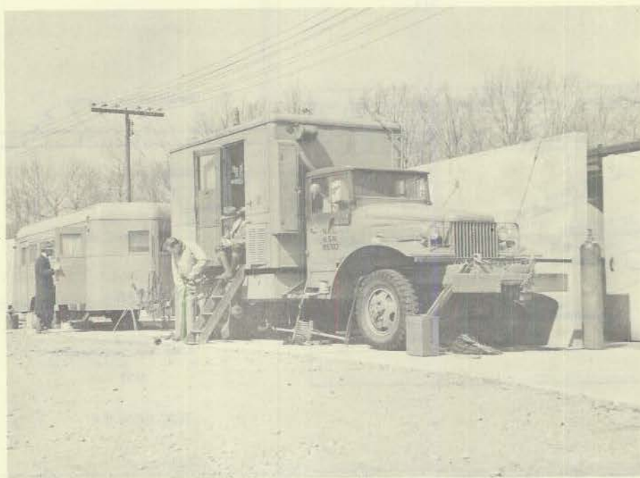
Fig. 10 - Truck-Trailer Laboratories and Protective Blast Wall
