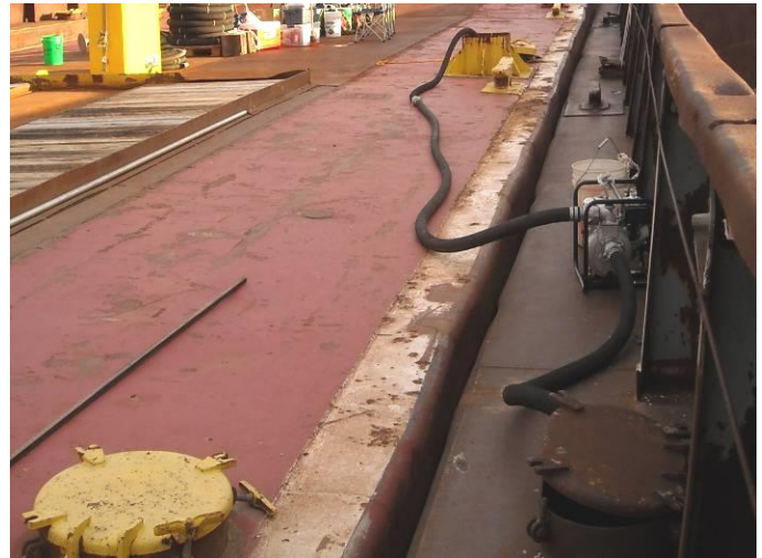
Pump and hose setup
