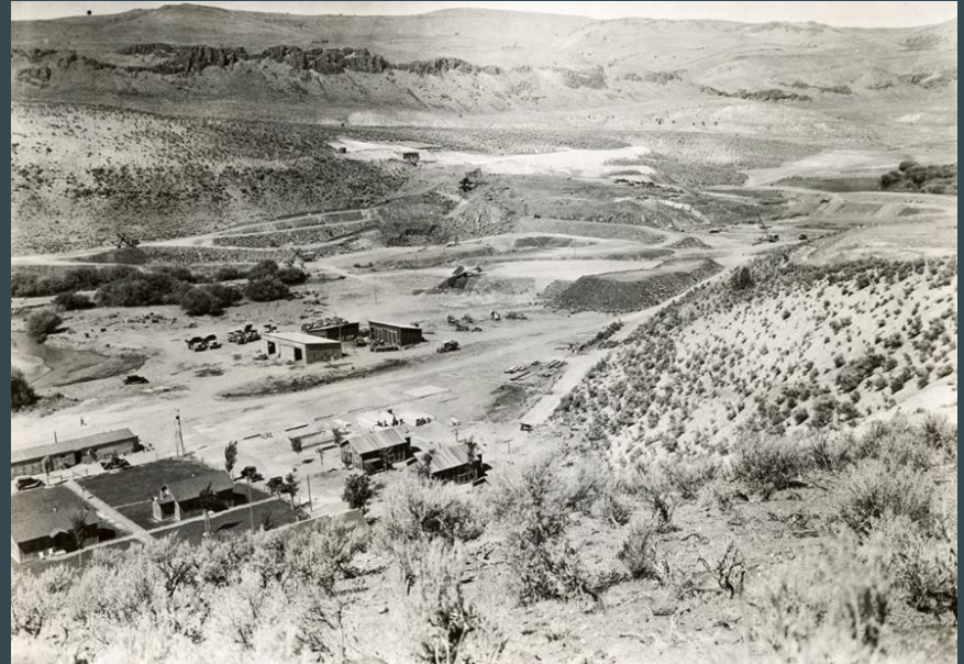
Construction of Agency Valley Dam (Oregon Historical Society)
