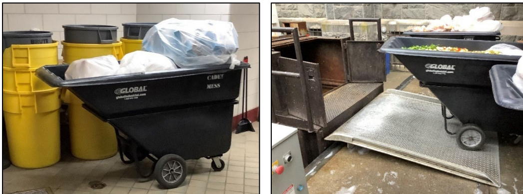
Figure 16. Left , full tilt truck ready for the compactor; right , Full tilt trucks about to be unloaded into the solid waste compactor at West Point's Cadet mess hall.
