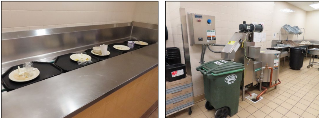
Figure 12. Left , tray return area from the diner's point of view; right , pulper and food waste only bin in the Raptor's Nest (JBLM) Clipper Room.
