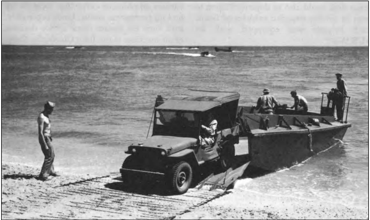
Figure 1. Army Engineers Training with Sommerfeld Matting at Camp Edwards Massachusetts
