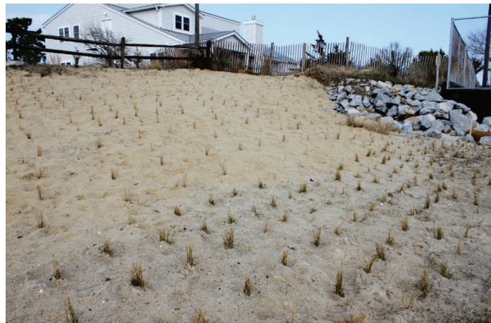
Figure 12. Photo showing project area immediately after planting occurred in April 2018. (Photo credit: Michael T. Boyle.)
