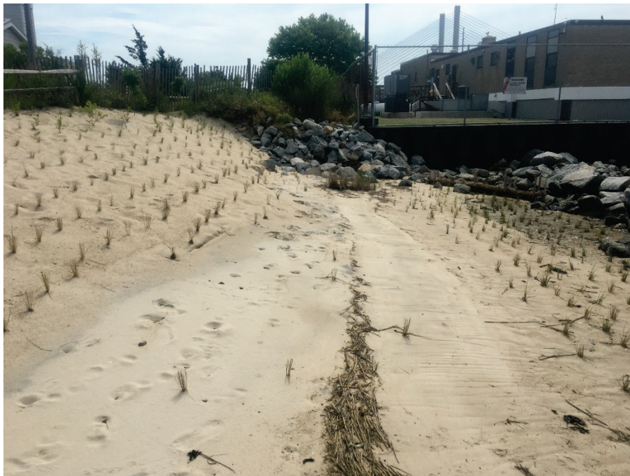
Figure 16. Midbeach loss of plants as of June 2018. Erosion observed in the midsection. (Photo credit: Bob Collins.)
