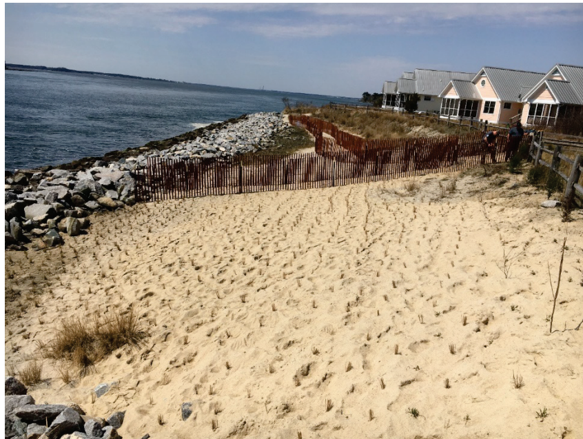
Figure 14. Planted area with protective fence installed on edges, serving as walking path. (Photo credit: Bob Collins.)
