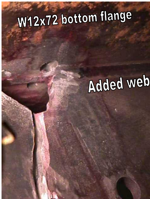
Figure 11-18: Crack faces arc-gouged and crack tips drilled.
