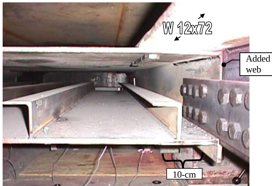
Figure 11-24: Tight clearances for bolting splice plates.
