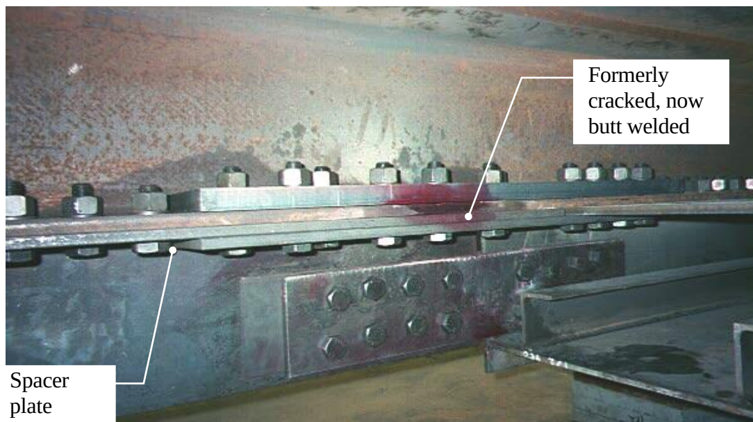
Figure 11-38: Final repair of cracked beam tension flange.
