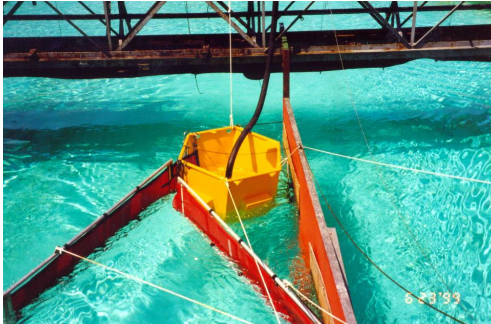
Figure 22. Circus Hull with Sweeping Arms Positioned near the Top of Hull.
