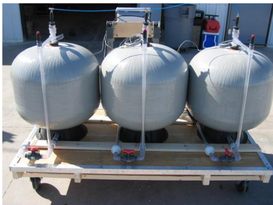
Figure 12. Thirty-gallon pressurized injection vessels for surrogates.
