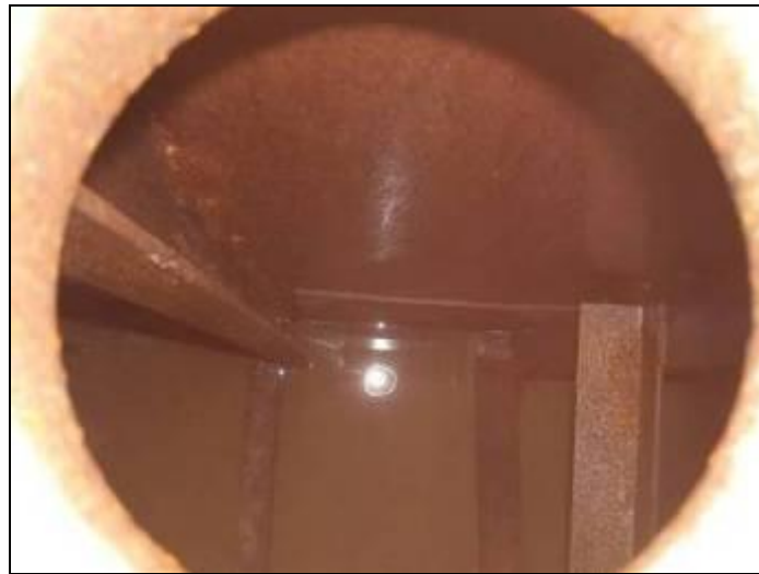
Figure 8. Typical tank inspection view.
