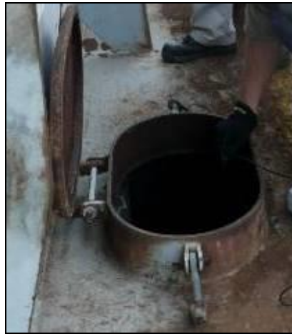
Figure 5. Ballast tank hinged manhole hatch.
