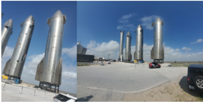
Figure 2. SpaceX Launch Facility Brownsville, TX 80
