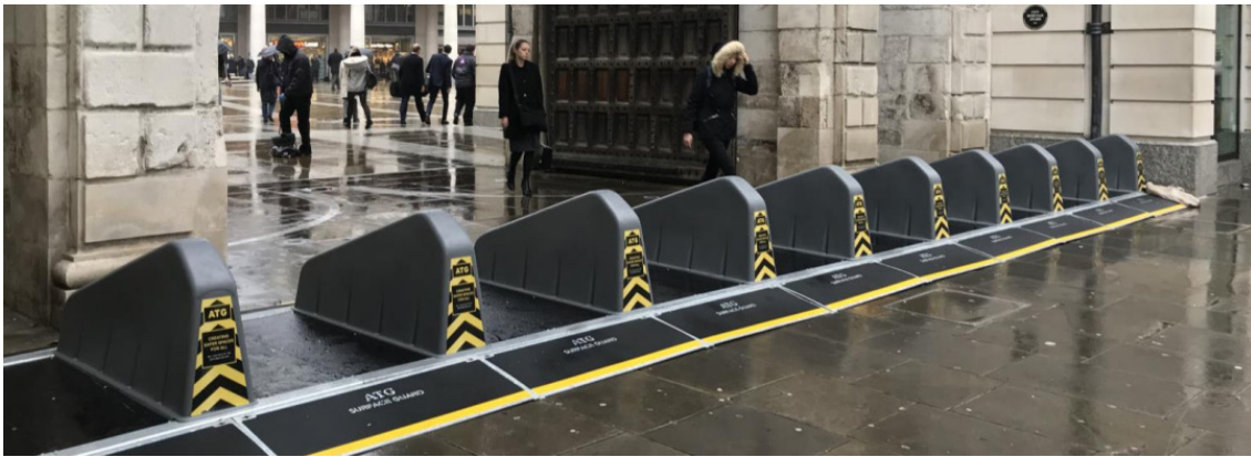
Figure 16. Surface Guard Barrier 181
