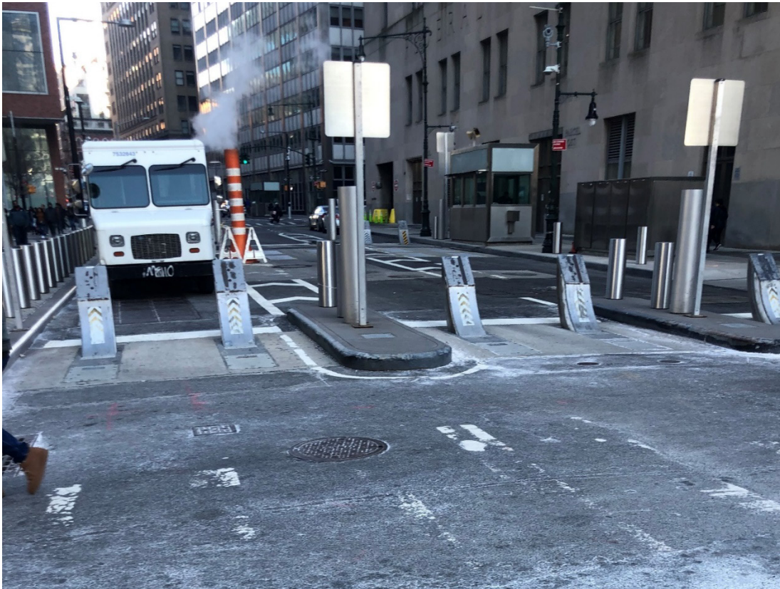
Figure 4. Permanent VSB Near the WTC Site
