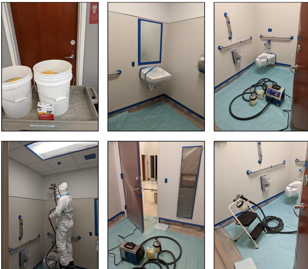
Figure 4. Demonstration area surface preparation and treatment with TPX-HL. Surfaces in each restroom were cleaned with trisodium phosphate solution (TSP) ( top left ). Masking off of all surfaces not to be treated is shown in the top middle and top right images. Application of photocatalytic coating to walls and ceiling with a high-pressure, low-volume (HPLV) sprayer ( bottom left ) and area after application ( bottom middle and right ).
