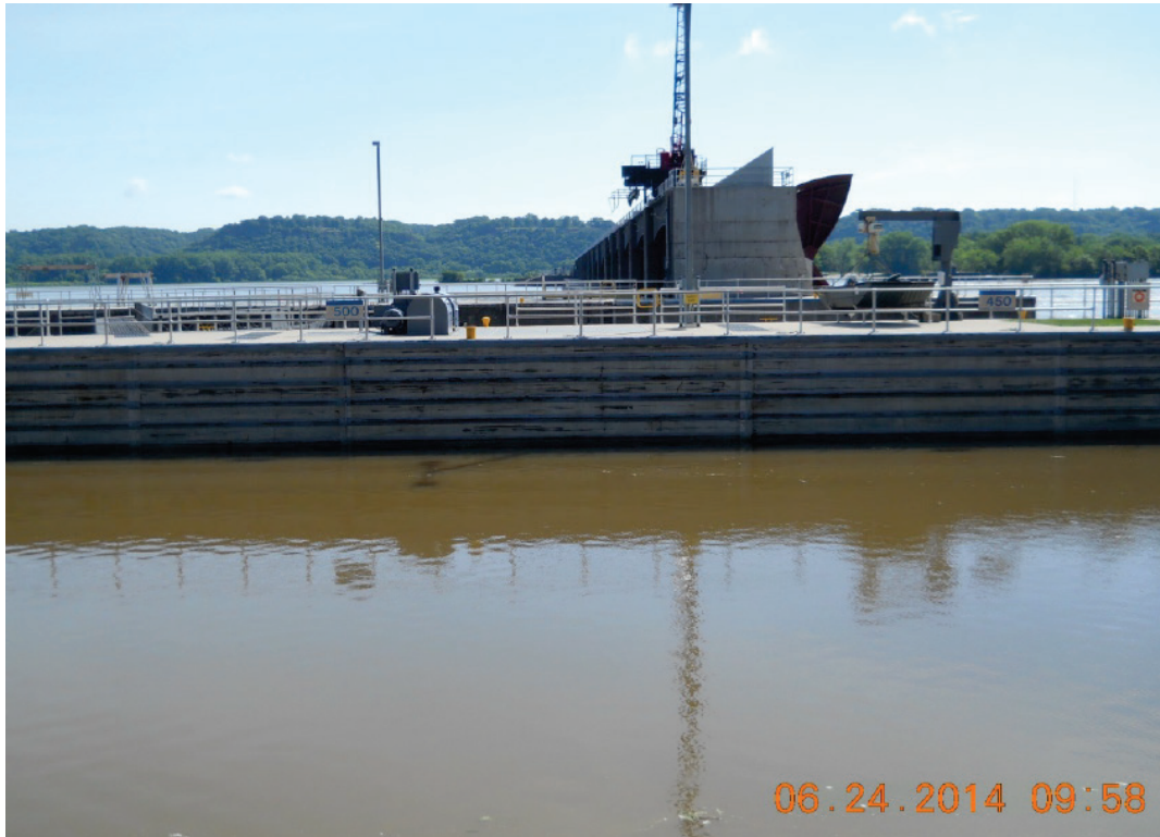
Figure 12. Lock 11—Precast panel repair in 2014.
