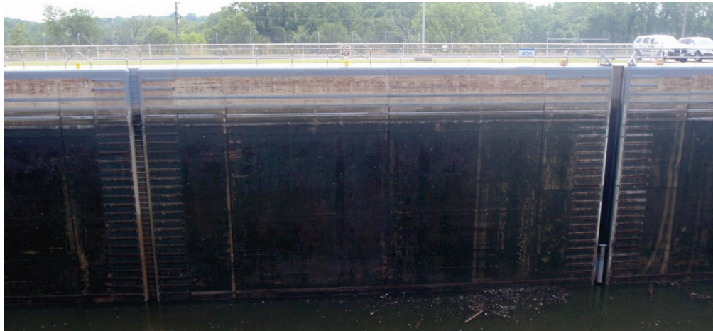
Figure 8. Lockport Lock CIP repair concrete in 2010.
