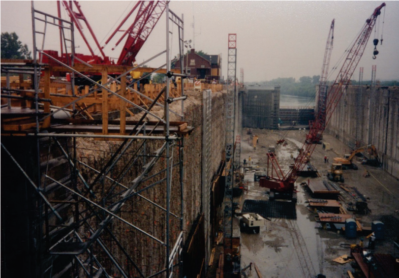
Figure 6. Lockport Lock wall during repair.
