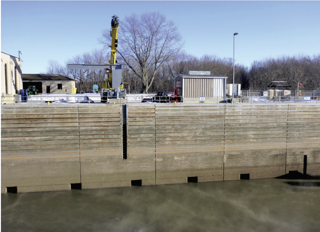
Figure 4. Lock 13—Cast-in-place concrete repair in winter 2016.
