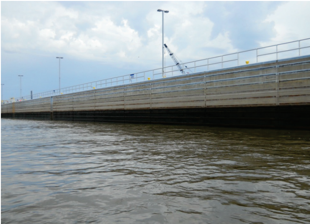
Figure 11. Lock 12—Precast panel repair in 2014.
