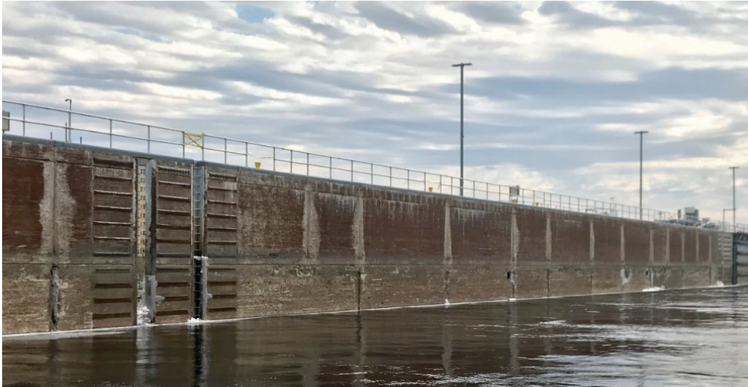
Figure 2. Lock 22 precast panels in February 2018.
