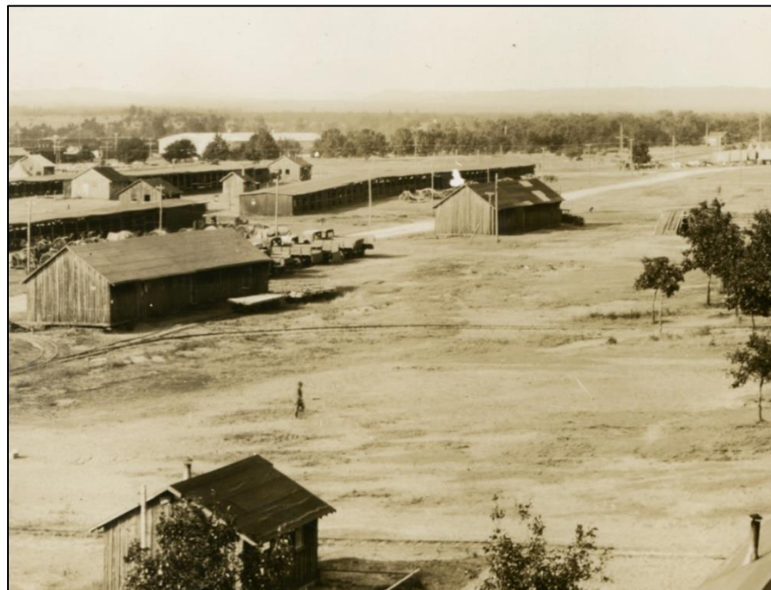
Figure 141. Narrow-gauge track branches from a frame storehouse at Camp McCoy in 1927. (Image from Monroe County Local History Room. Public domain.) 374
