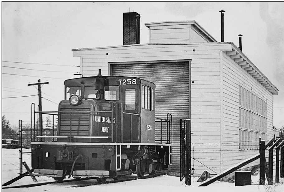
Figure 47. Diesel switch engine 7258 is seen outside the engine house (2163, not extant) in 1952. Looking north. (Image from Monroe County Local History Room. Public domain.) 213
