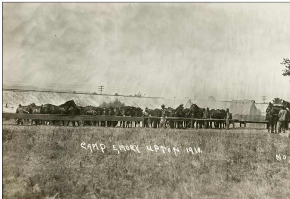
Figure 25. Another view of the railroad grade near Camp Emory Upton, 1910. Note the elevation of the tracks and the sandy composition of the bed. (Image from Monroe County Local History Room. Public domain.) 132
