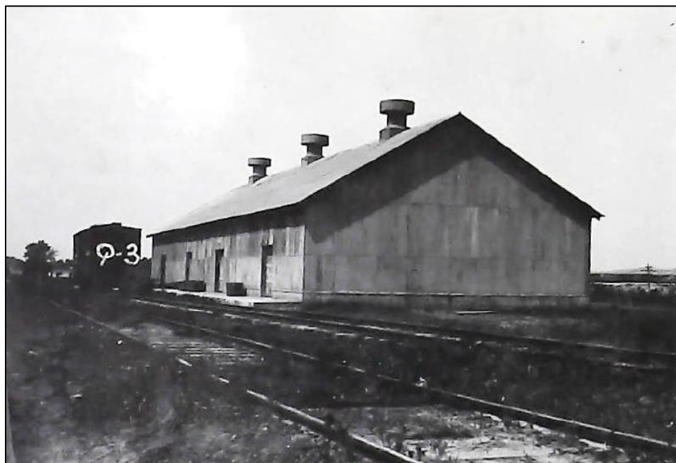
Figure 94. A 120 x 40 ft galvanized iron warehouse constructed at Camp Emory Upton, c. 1910. Image taken after its relocation to Camp Robinson in 1928. (Image from Fort McCoy CRM. Public domain.) 295
