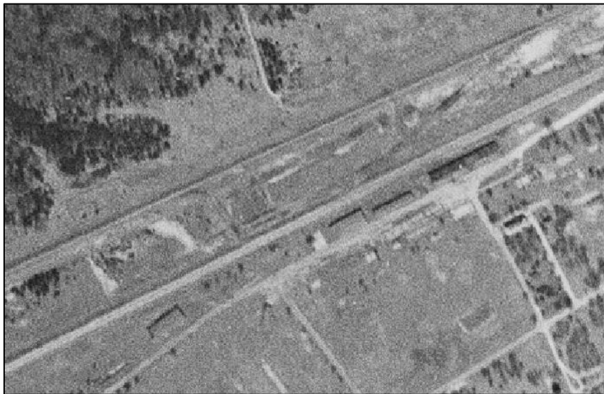
Figure 117. A 1958 aerial photograph shows that the depots at McCoy Station West had been demolished. (Image from USGS Earth Explorer. Public domain.) 329
