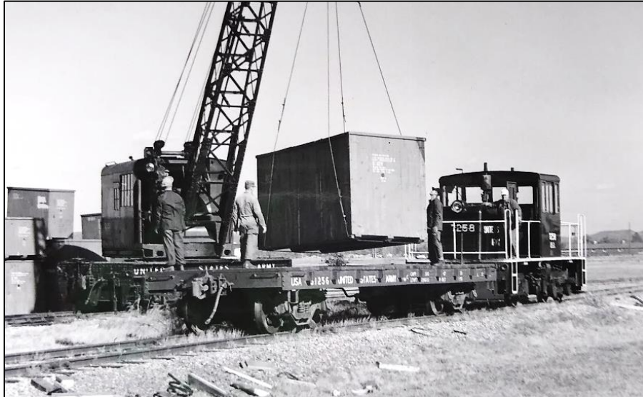
Figure 41. A crane hoists a five-ton crate from an Army flatbed car in 1950. (Image from NARA. Public domain.) 206
