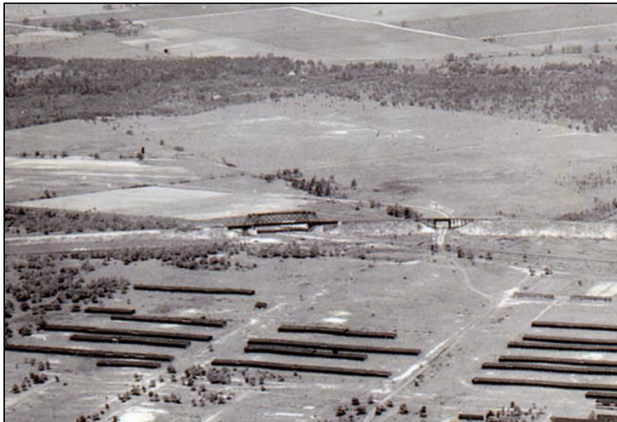
Figure 165. The C&NW truss bridge as seen from the air, c. 1925. Looking west. (Image from Monroe County Local History Room. Public domain.) 457
