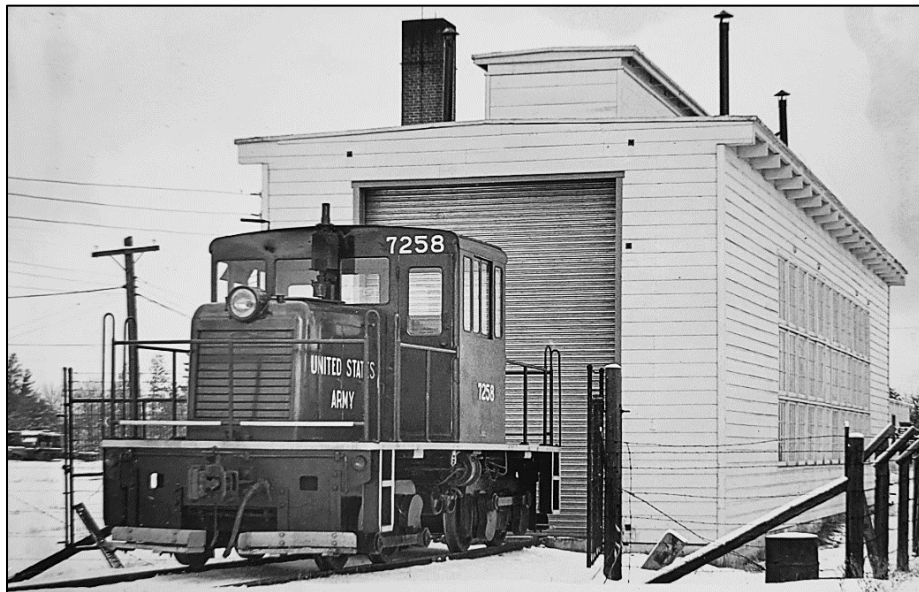
Figure 151. A diesel switch engine is seen outside the engine house (2163) in 1952, looking northwest. (Image from Monroe County Local History Room. Public domain.) 421
