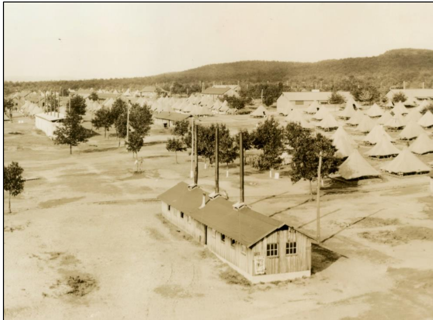
Figure 140. Two sets of narrow-gauge track wend past tents at Camp McCoy in 1927. (Image from Monroe County Local History Room. Public domain.) 373
