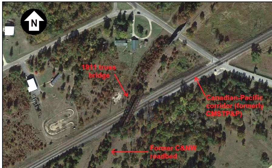
Figure 164. Satellite view of the abandoned C&NW truss bridge. (Map data: Google, 2013.)
