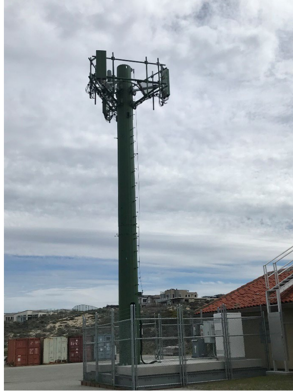
Figure 7. AT&T 5G 50-ft Millimeter Wave Tower. Source: LCDR Caplan iPhone (2022).
