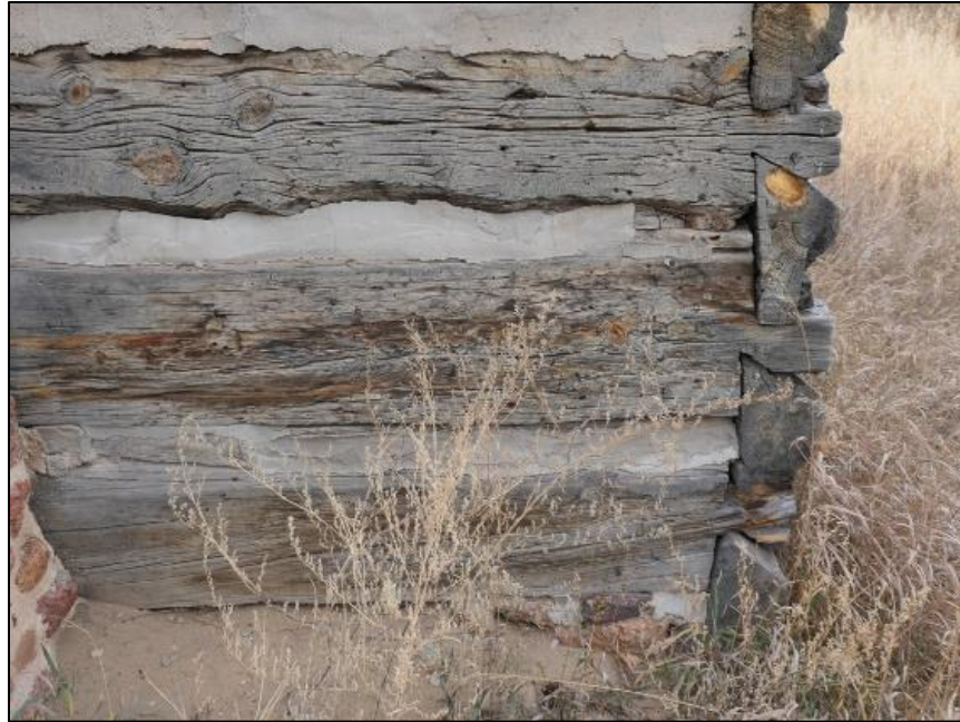
Figure 44. Looking at exterior logs and connections at the lower northeast corner of the Burgess-Capps Cabin (photo by ERDC-CERL researchers, 2021).
