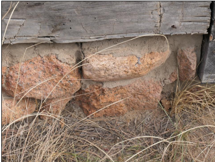
Figure 67. Mortar along with the stone foundation of the Burgess-Capps Cabin (photo by ERDC-CERL researchers, 2021).
