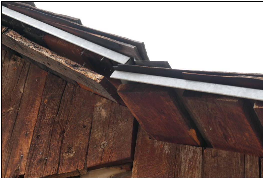
Figure 82. Galvanized metal edging along the board edges of the porch roof on the west side of the Burgess-Capps Cabin (photo by ERDC-CERL researchers, 2021).
