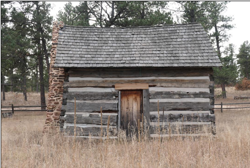
Figure 24. Looking south at the north side of the Burgess-Capps Cabin (photo by ERDC-CERL researchers, 2021).
