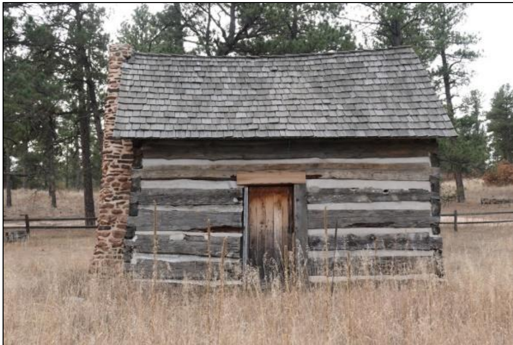
Figure 32. Looking at the wood wall, trim, and roof details of the south elevation of the Burgess-Capps Cabin (photo by ERDC-CERL researchers, 2021).
