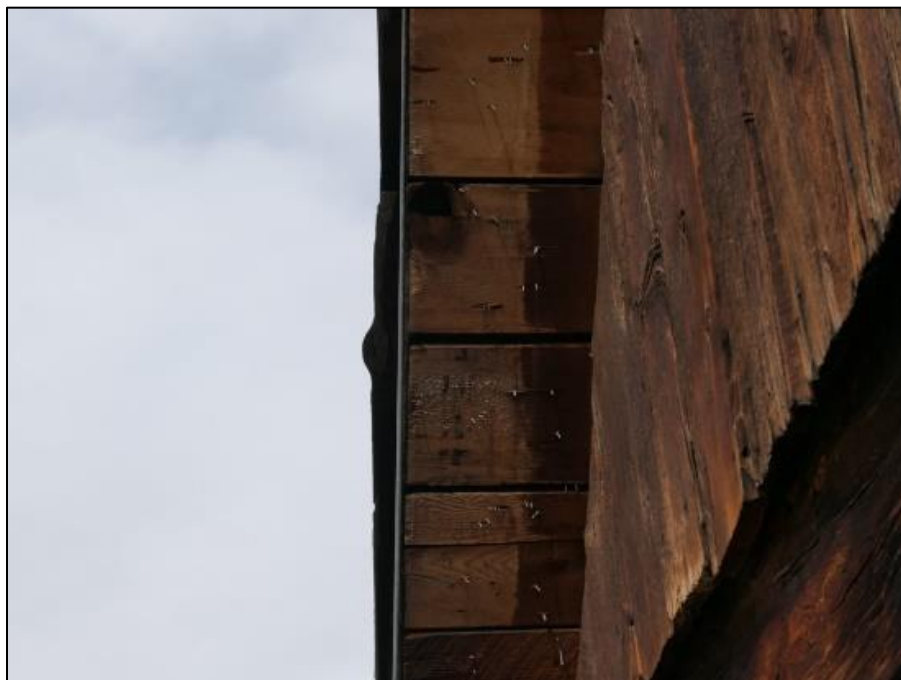
Figure 36. Looking at wood soffits and vertical siding along the gable of the Burgess-Capps Cabin (photo by ERDC-CERL researchers, 2021).
