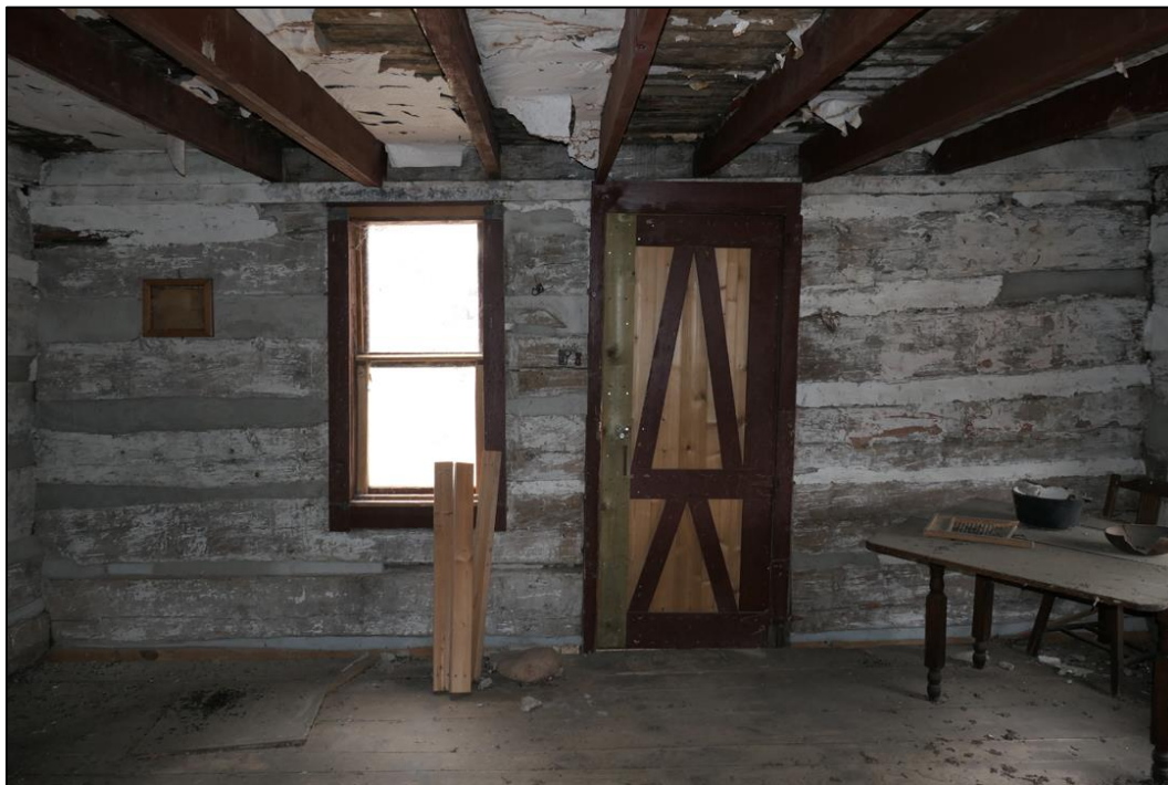
Figure 28. Looking at the south interior wall on the first floor of the Burgess-Capps Cabin (photo by ERDC-CERL researchers, 2021).
