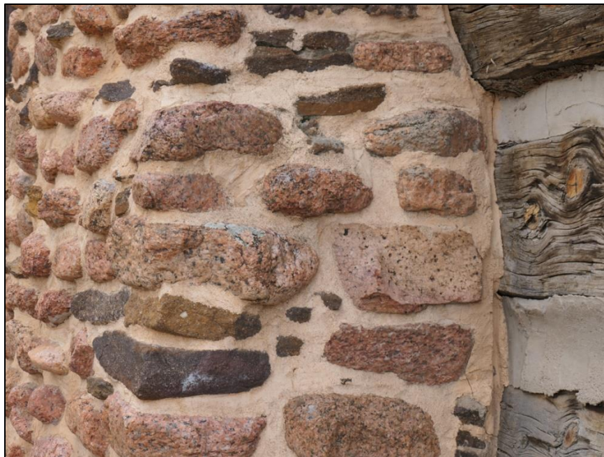
Figure 74. Multiple stone sizes on the chimney of the Burgess-Capps Cabin (photo by ERDC-CERL researchers, 2021).
