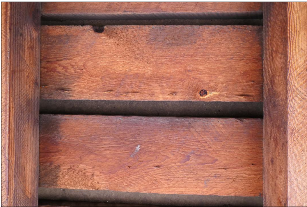
Figure 47. Wood planks that make up the porch roof of the Burgess-Capps Cabin (photo by ERDC-CERL researchers, 2021).
