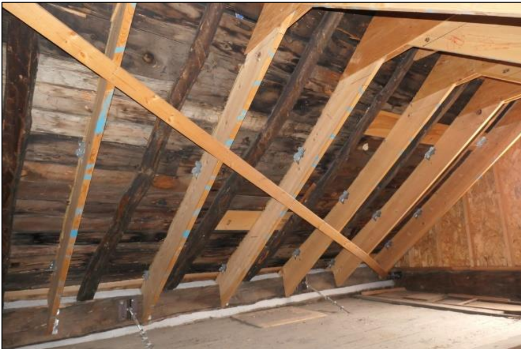
Figure 61. Wood structural reinforcements added to the roof of the Burgess-Capps Cabin at an unknown date (i.e., no documentation found) (photo by ERDC-CERL researchers, 2021).
