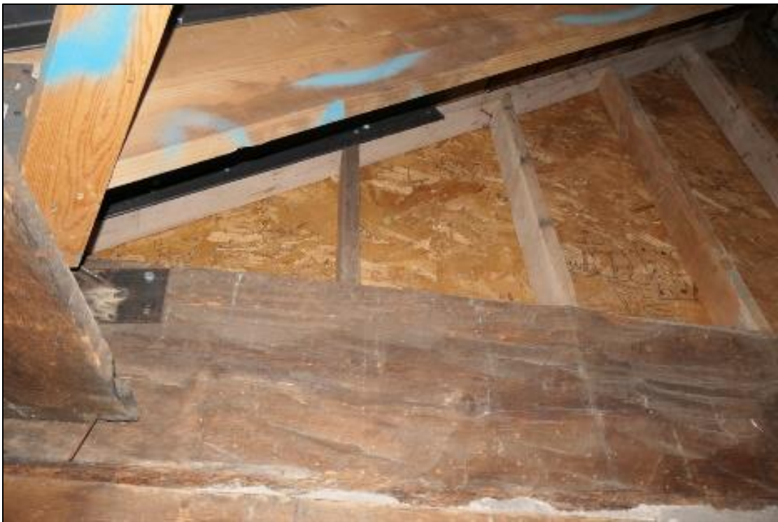
Figure 60. Wood structural reinforcements added to the gables of the Burgess-Capps Cabin at an unknown date (i.e., no documentation found) (photo by ERDC-CERL researchers, 2021).
