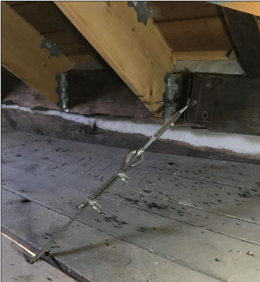
Figure 119. Close-up of a cable, turnbuckle, and bracket used to tie the loft floor joists to a wall top timber (photo by ERDC-CERL researchers, 2021).
