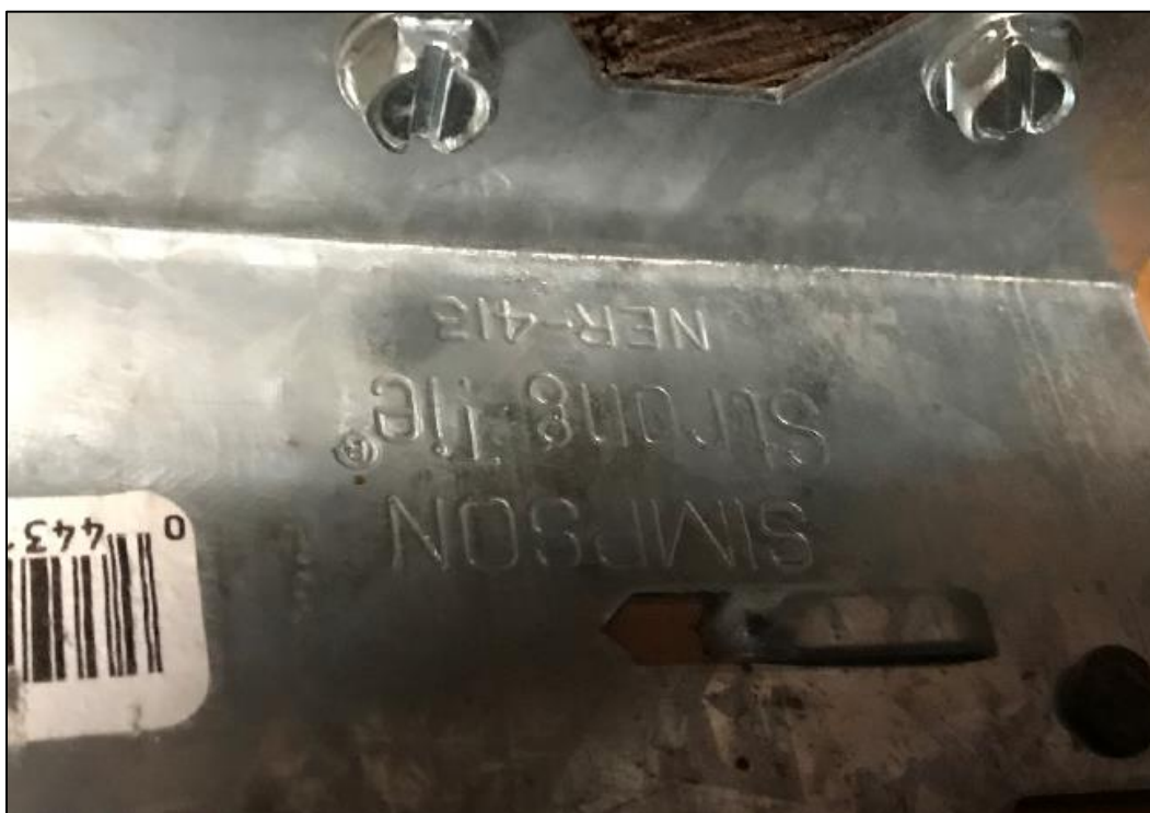
Figure 116. Simpson Strong-tie NER-413 metal brackets used to anchor the roof boards to the new joists (photo by ERDC-CERL researchers, 2021).
