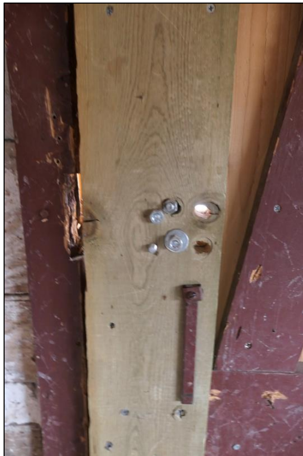
Figure 87. Various types of metal hardware on the interior side of the door of the Burgess-Capps Cabin (photo by ERDC-CERL researchers, 2021).
