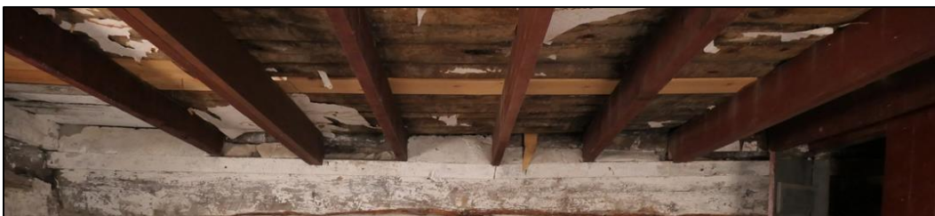
Figure 63. Floor joists below the loft floor (photo by ERDC-CERL researchers, 2021).
