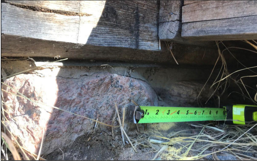
Figure 83. Looking at galvanized metal flashing on the top of the stone foundation of the Burgess-Capps Cabin (photo by ERDC-CERL researchers, 2021).
