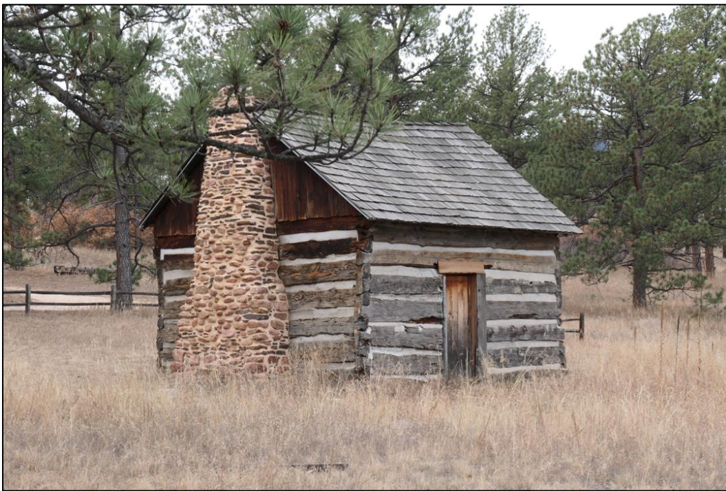
Figure 25. Looking southwest at the Burgess-Capps Cabin (photo by ERDC-CERL researchers, 2021).
