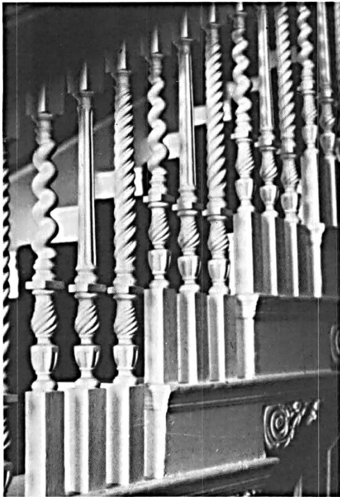
Do not Abrasively Clean these Interiors. Most historic residential and some commercial interior spaces contain finished plaster and wooden elements such as this stair balustrade and paneling which contribute to the historic and architectural character of the structure. Such interiors should not be subjected to abrasive techniques for the purpose of removing paint, dirt, discoloration or plaster.
