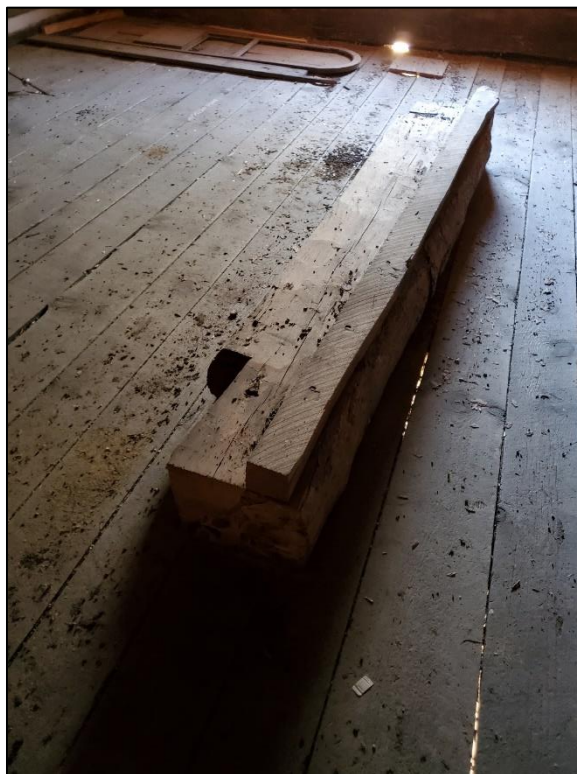
Figure 152. Timber found in the attic that appears cut to fit as a header over the north doorway (photo by ERDC-CERL researchers, 2021).
