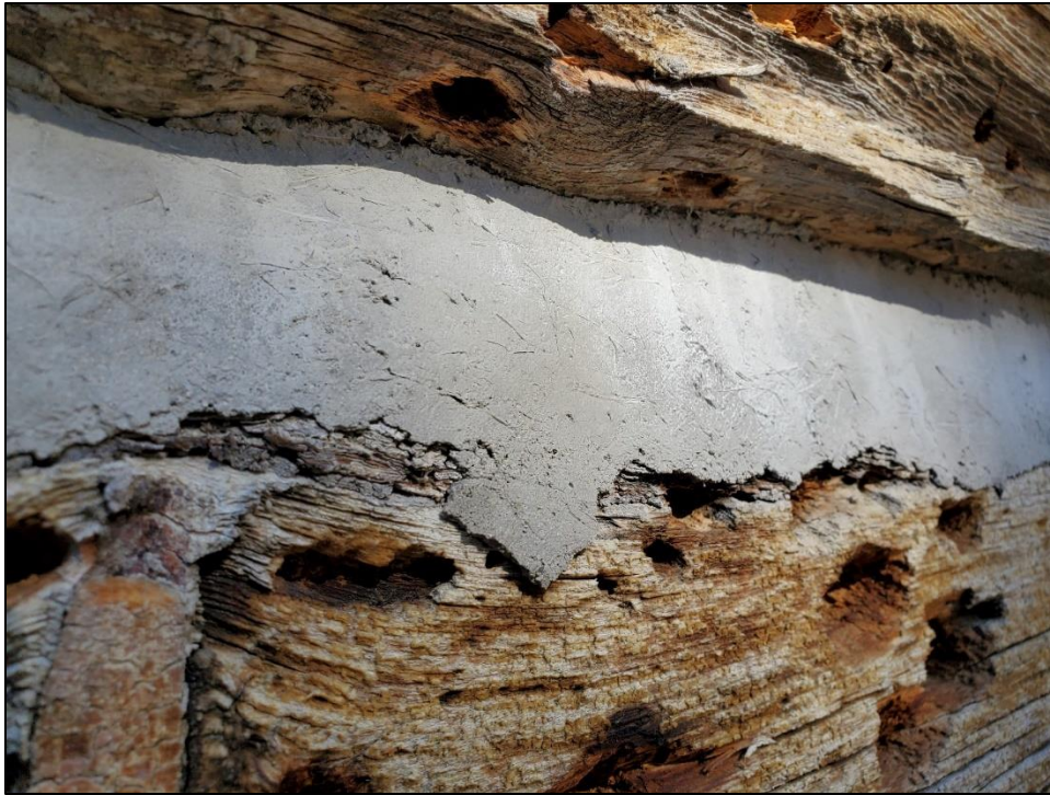
Figure 161. Typical rough surface finish resulting from fibers in fiber-reinforced mortar.
