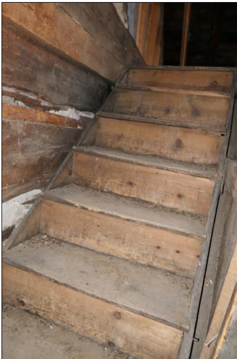
Figure 54. Interior view of the wooden stairwell leading to the loft of the Burgess-Capps Cabin (photo by ERDC-CERL researchers, 2021).
