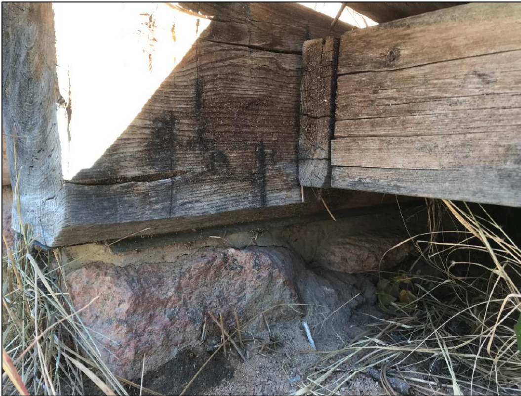
Figure 98. Stone and mortar foundation at the west end of the south wall (photo by ERDC-CERL researchers, 2021).
