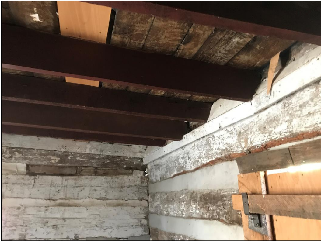
Figure 112. Floor joists below the loft floor (photo by ERDC-CERL researchers, 2021).
