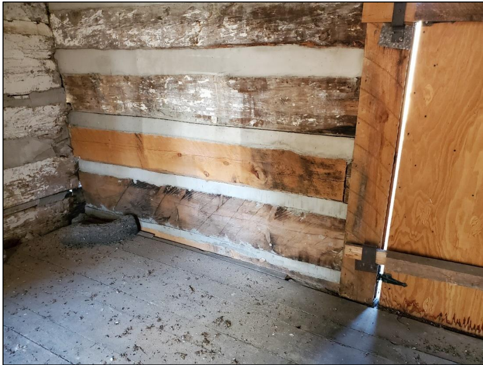
Figure 155. Freshly sawn timber in the north interior wall (sample 14) (photo by ERDC-CERL researchers, 2021).
