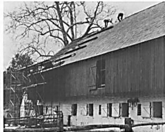
11. The replacement sawn red cedar shingles matched the deteriorated shingles exactly for this barn re-roofing. The old shingles, seen to the far left, were removed as the new shingles were installed. Even the horizontal coursing matched because the exposure length for both old and new shingles was the same. Photo: Williamsport Preservation Training Center.
