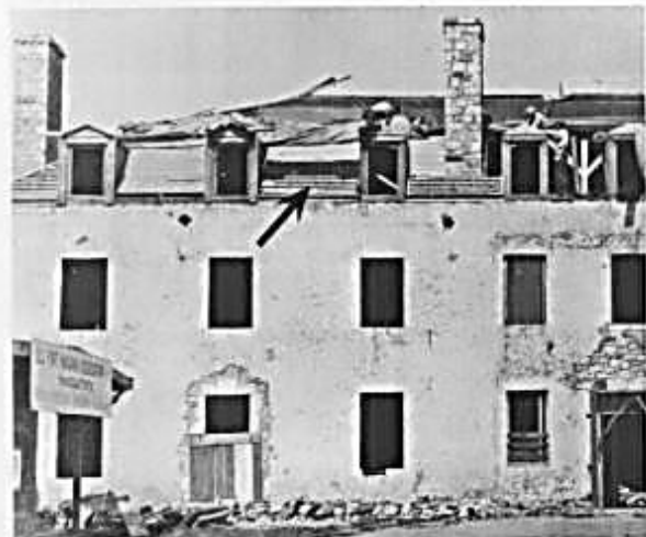
9. This 1927 view of the reshingling of the French Castle at Old Fort Niagara, N.Y., shows the wooden sleepers being laid (see arrow) over solid sheathing in order to raise the shingles up slightly to allow under-shingle ventilation. Note that the horizontal strips are not continuous to allow airflow and trapped moisture to drain away. This cedar roof has lasted for over 60 years in a harsh moist environment. Photo: Old Fort Niagara, Assoc. Inc.
