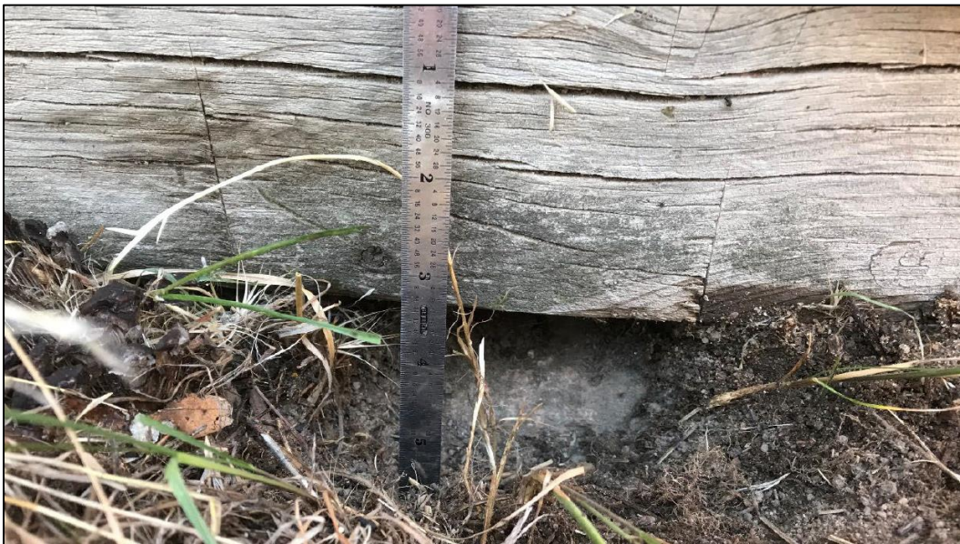
Figure 101. Foundation below the east wall, near the south wall, where mortar and possibly stone is below the lowest timber (photo by ERDC-CERL researchers, 2021).
