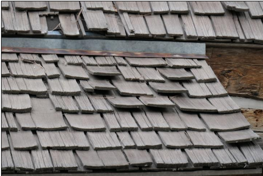
Figure 33. Looking at wood shingles at the meeting point of the roof and porch roof on the south side of the Burgess-Capps Cabin (photo by ERDC-CERL researchers, 2021).
