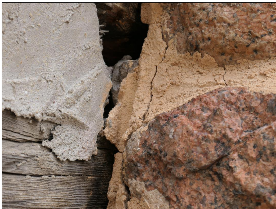
Figure 69. Mortar color difference between log and stone mortar (photo by ERDC-CERL researchers, 2021).
