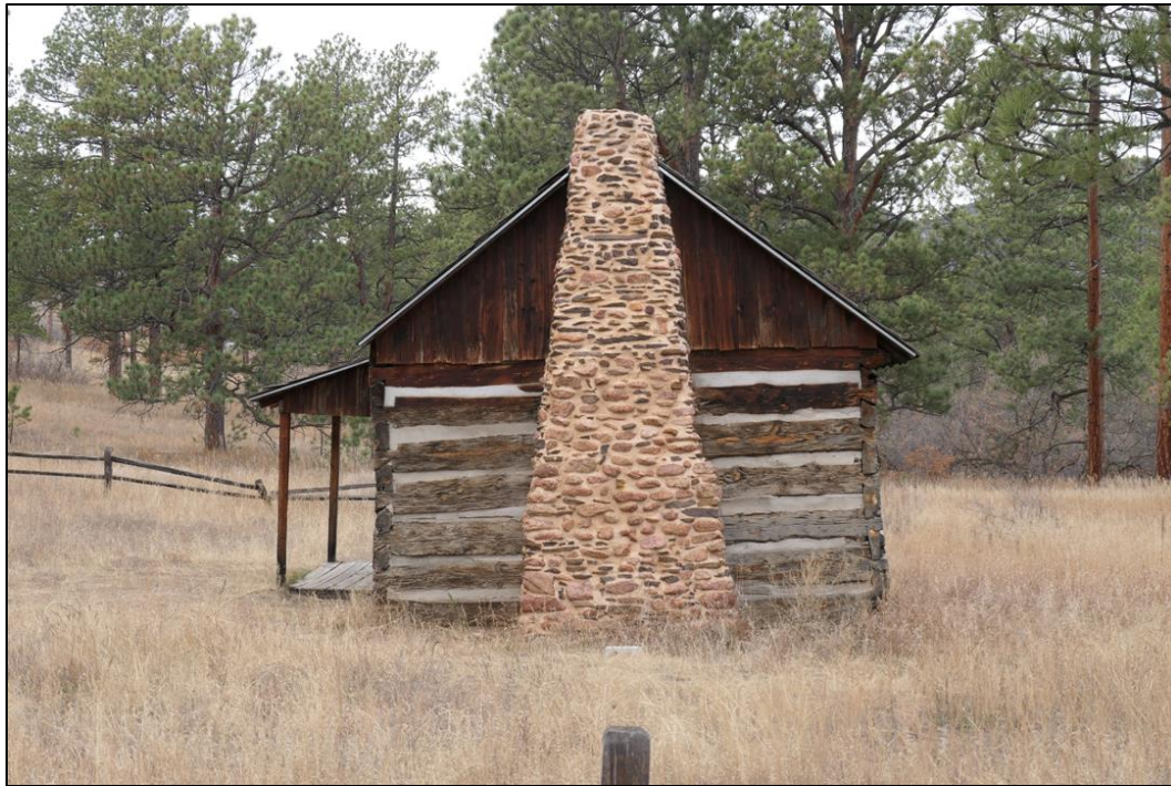
Figure 72. Front view of the stone chimney on the east elevation of the Burgess-Capps Cabin (photo by ERDC-CERL researchers, 2021).
