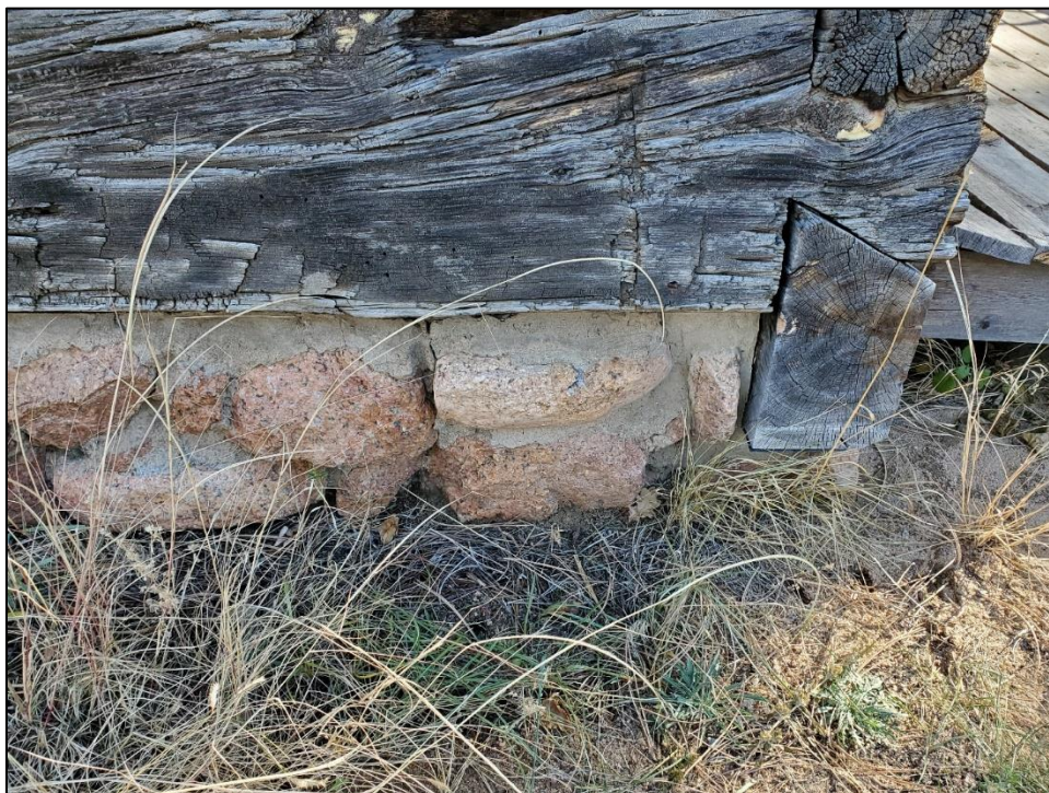
Figure 160. Example interface between the stone foundation and the west wall timbers (photo by ERDC-CERL researchers, 2021).
