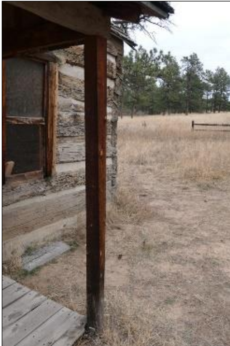
Figure 45. Wood 4 × 4 supporting the porch roof of the Burgess-Capps Cabin (photo by ERDC-CERL researchers, 2021).
