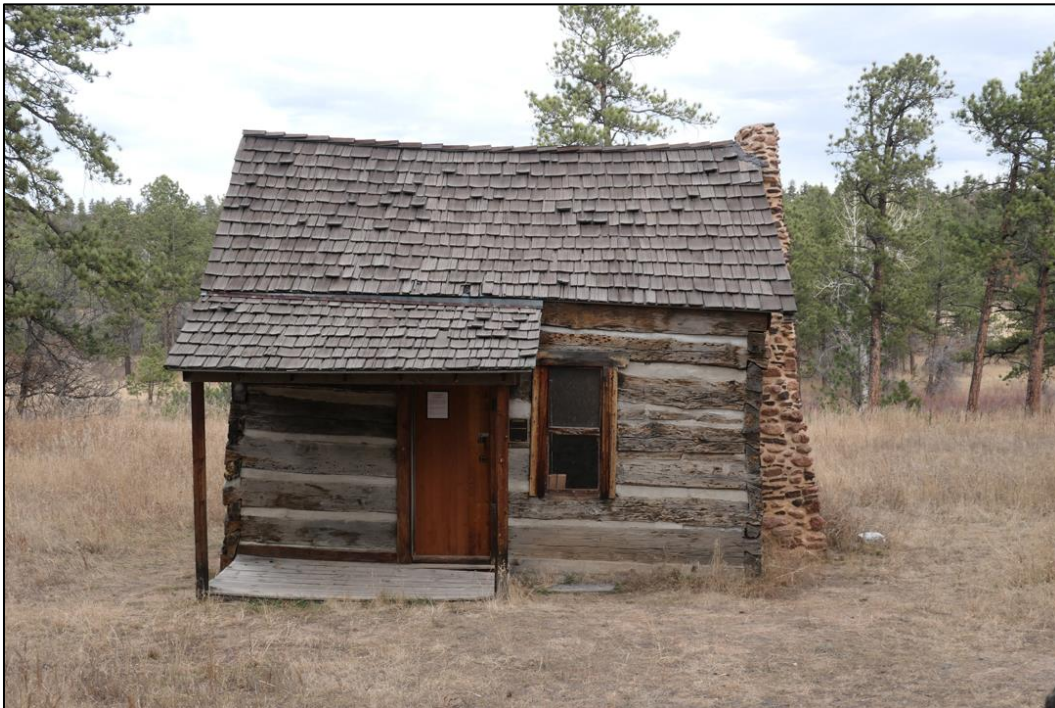
Figure 64. Overall look at exterior mortar composition on the south elevation of the Burgess-Capps Cabin (photo by ERDC-CERL researchers, 2021).
