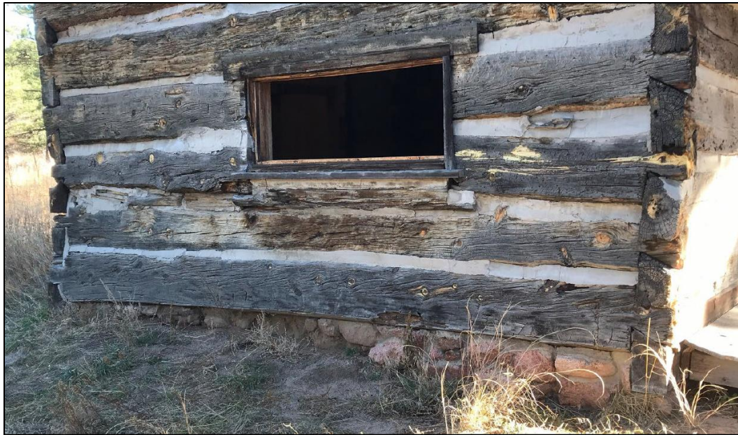
Figure 97. Stone and mortar foundation at the west wall (photo by ERDC-CERL researchers, 2021).
