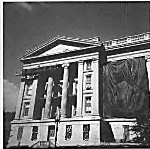
Figure 23. A tarpaulin protects and shields pedestrians from potentially harmful spray while chemical cleaning is underway on the granite exterior of the U.S. Treasury Building, Washington, D.C.
