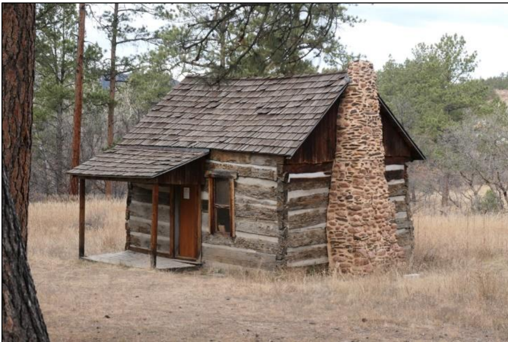
Figure 20. Looking northwest at the Burgess-Capps Cabin (photo by ERDC-CERL researchers, 2021).
