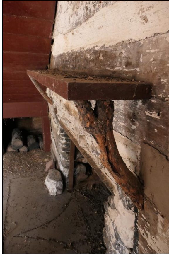
Figure 59. Wood mantle and wood-stick posts above the fireplace in the Burgess-Capps Cabin (photo by ERDC-CERL researchers, 2021).
