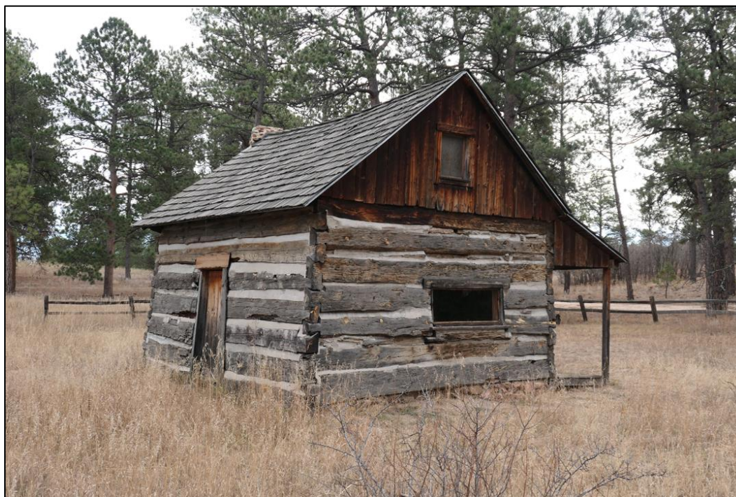
Figure 23. Looking southeast at the Burgess-Capps Cabin (photo by ERDC-CERL researchers, 2021).
