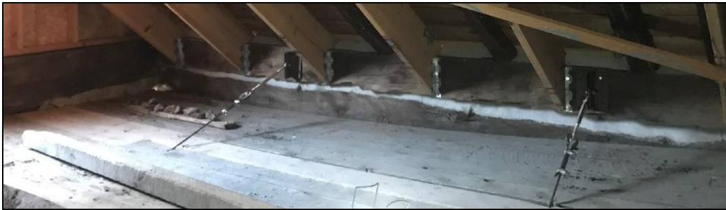
Figure 111. Loft floor joist with the turnbuckles and threaded rods running to the top of the wall timbers (photo by ERDC-CERL researchers, 2021).
