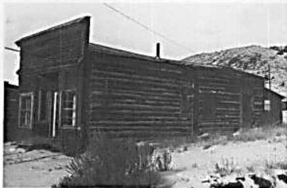
Fig. 4. Beginning around the mid-19th century, entire western boomtowns were hastily constructed of frame and log, such as the buildings in Bannack, Montana, the site of the State's first gold discovery. Photo: National Park Service Files.
