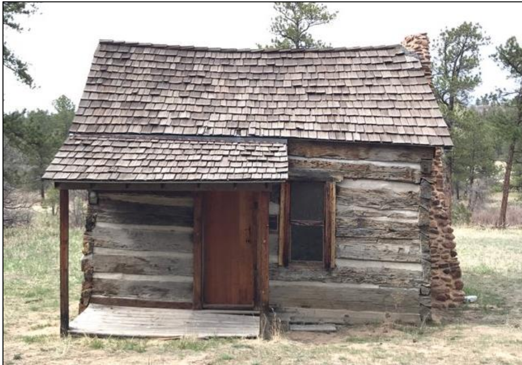
Figure 95. Front-exterior (south side) view of the log cabin (photo by ERDC-CERL researchers, 2021).
