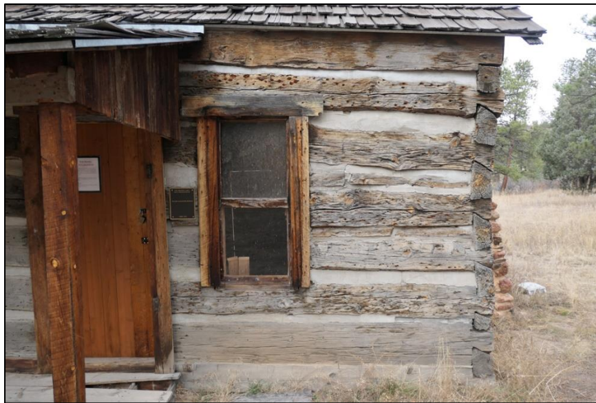
Figure 42. Wooden window trim on the south elevation of the Burgess-Capps Cabin (photo by ERDC-CERL researchers, 2021).
