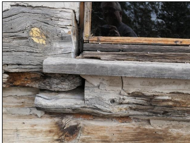
Figure 40. Looking at the connection of the exterior logs and wood windowsill on the west side of the Burgess-Capps Cabin (photo by ERDC-CERL researchers, 2021).
