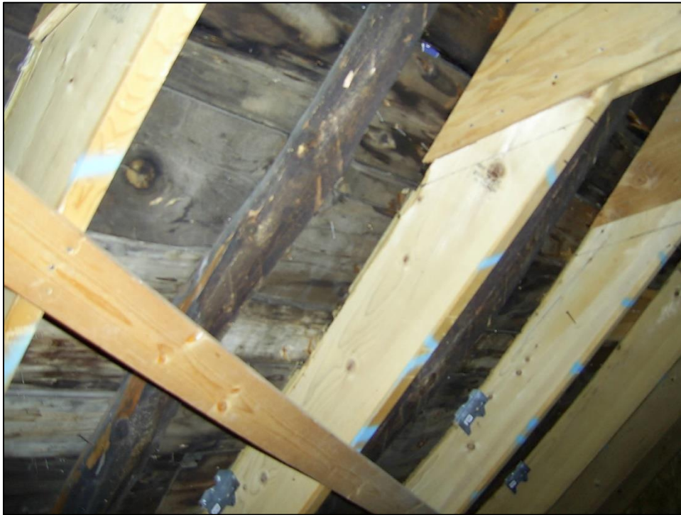
Figure 110. Wood joists added to one side of the roof without roof sheathing (photo by ERDC-CERL researchers, 2021).
