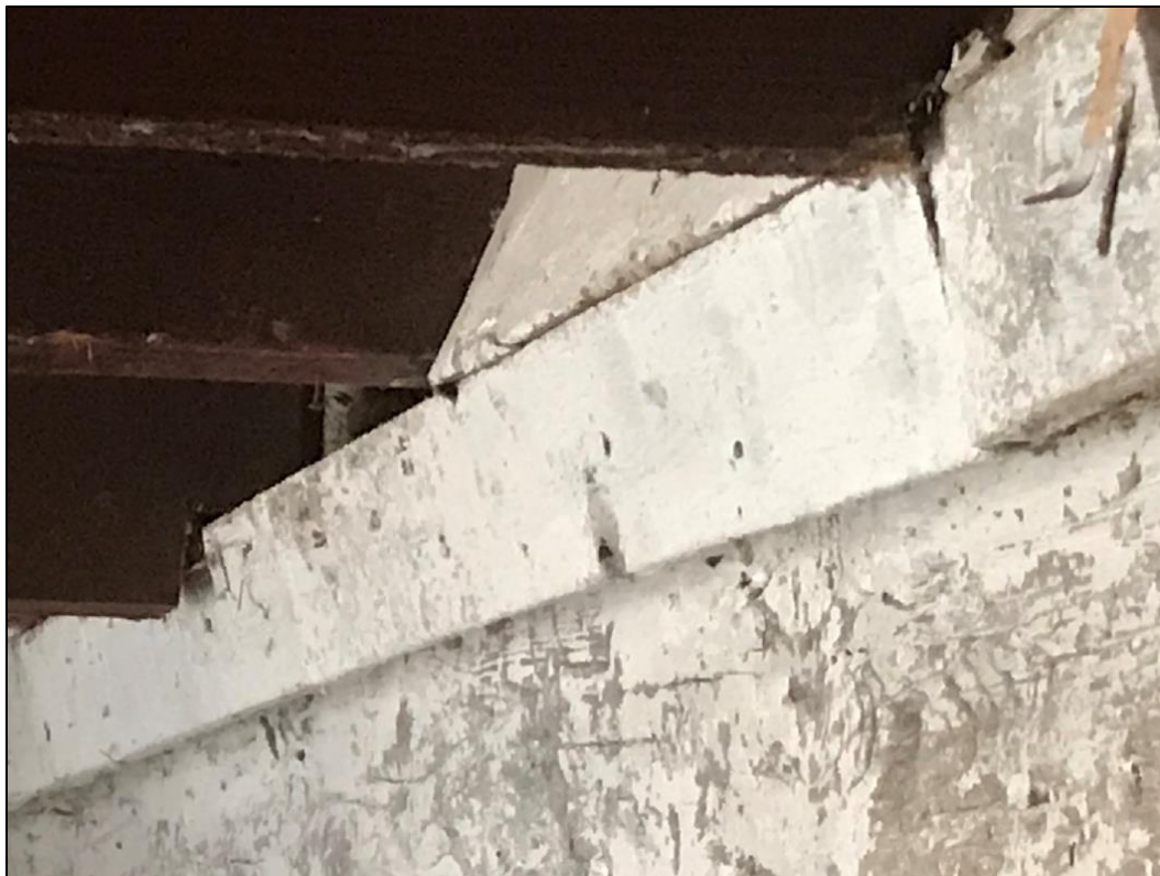
Figure 113. Closeup view of the joist-supporting 2 × 4 along the north wall (photo by ERDC-CERL researchers, 2021).
