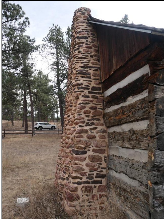
Figure 73. Side view of the stone chimney on the east elevation of the Burgess-Capps Cabin (photo by ERDC-CERL researchers, 2021).
