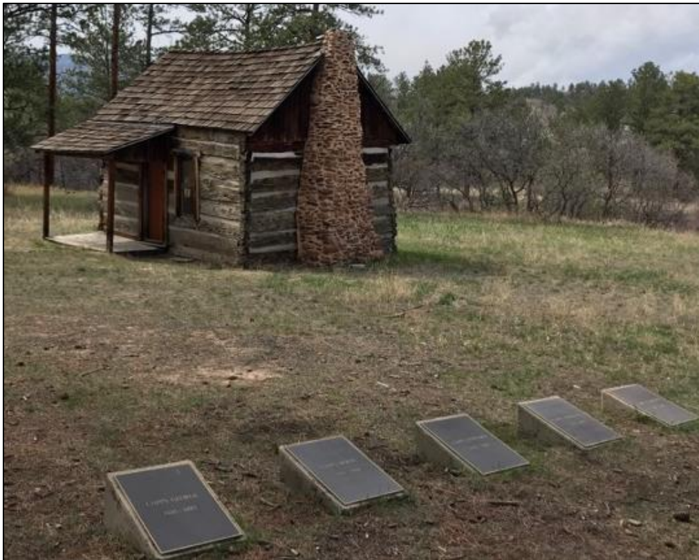
Figure 94. Exterior view of the log cabin and chimney from the southeast corner (photo by ERDC-CERL researchers, 2021).
