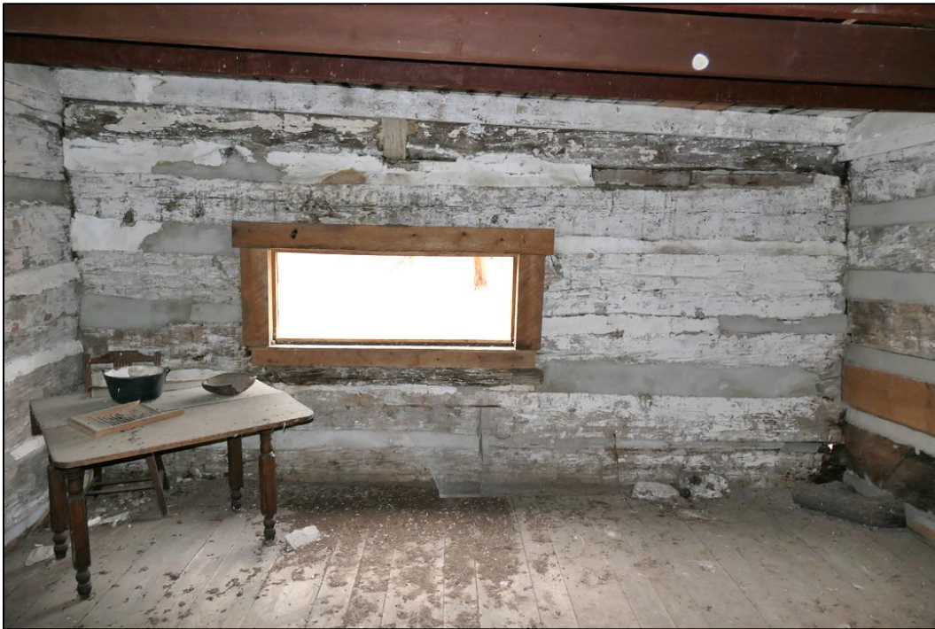
Figure 26. Looking at the west interior wall on the first floor of the Burgess-Capps Cabin (photo by ERDC-CERL researchers, 2021).
