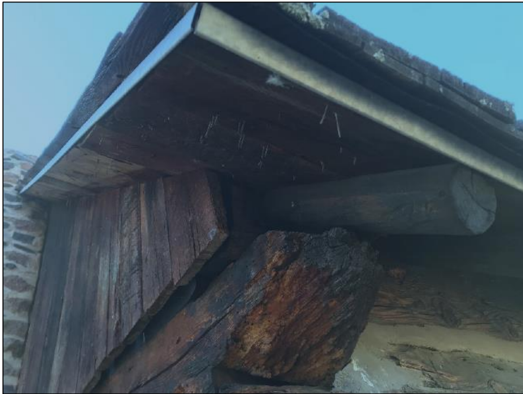
Figure 114. Exterior view of the northwest corner of the roof showing the roof boards, galvanized metal edge, old roof joist, and gable end wall planks (photo by ERDC-CERL researchers, 2021).
