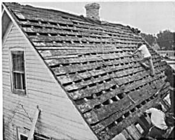
7. The reshingling of the circa 1856 Stovewood House in Decorah, Iowa, revealed the original open sheathing boards and pole rafters. Sawn cedar shingles were used as a replacement for the historic cedar shingles seen still in place at the ridge. A new starter course is being laid at the eaves. Photo: Norwegian-American Museum, Decorah, Iowa.
