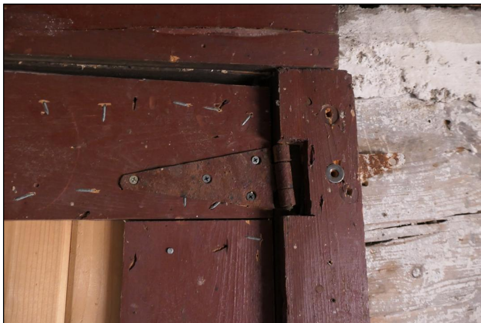
Figure 86. Metal hinge on a door in the Burgess-Capps Cabin (photo by ERDC-CERL researchers, 2021).
