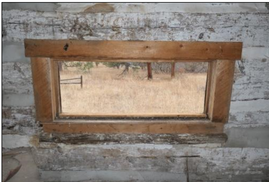
Figure 57. Interior wood window trim on the west wall of the Burgess-Capps Cabin (photo by ERDC-CERL researchers, 2021).
