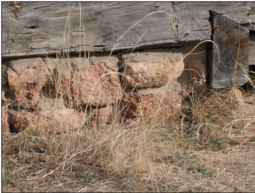
Figure 76. Stone foundation of the Burgess-Capps Cabin (photo by ERDC-CERL researchers, 2021).
