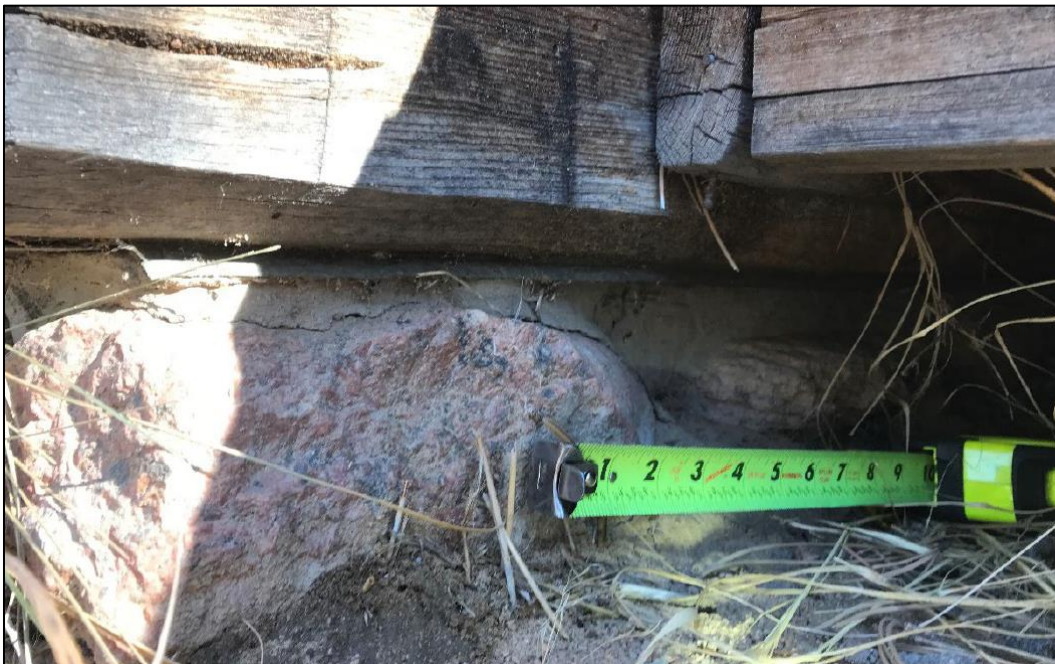
Figure 99. Closeup view of the foundation wall at the west end of the south wall showing galvanized metal flashing (photo by ERDC-CERL researchers, 2021).
