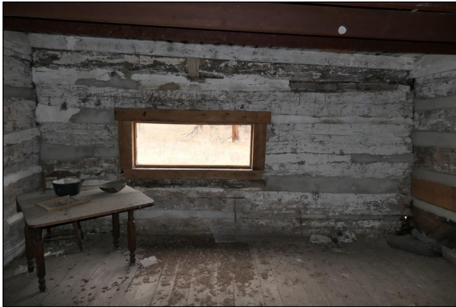
Figure 70. Overall look at the interior mortar composition on the west interior wall of the Burgess-Capps Cabin (photo by ERDC-CERL researchers, 2021).
