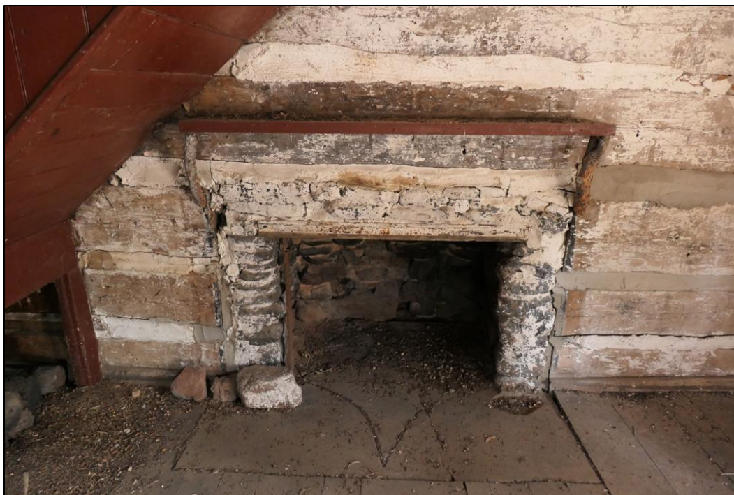
Figure 78. Stone fireplace on the interior east wall of the Burgess-Capps Cabin (photo by ERDC-CERL researchers, 2021).
