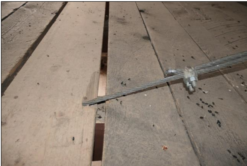
Figure 62. Wood loft floor, which is also the ceiling of the first floor at the Burgess-Capps Cabin (photo by ERDC-CERL researchers, 2021).
