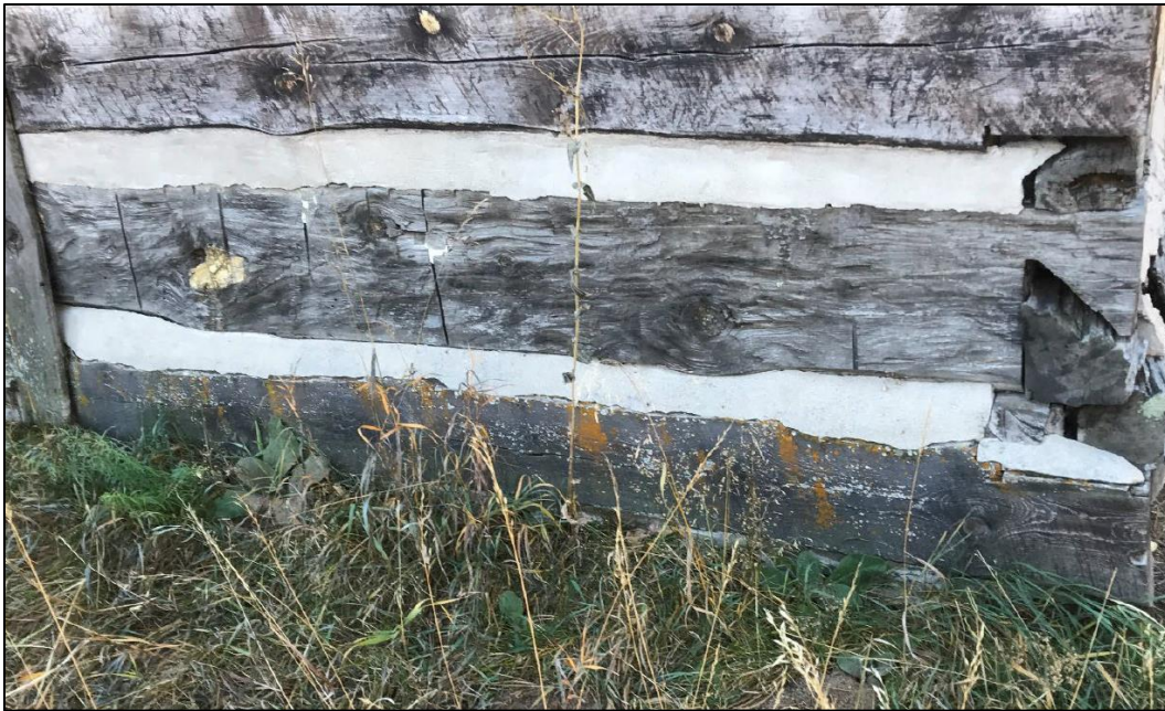
Figure 100. Foundation at the west end of the north wall (photo by ERDC-CERL researchers, 2021).
