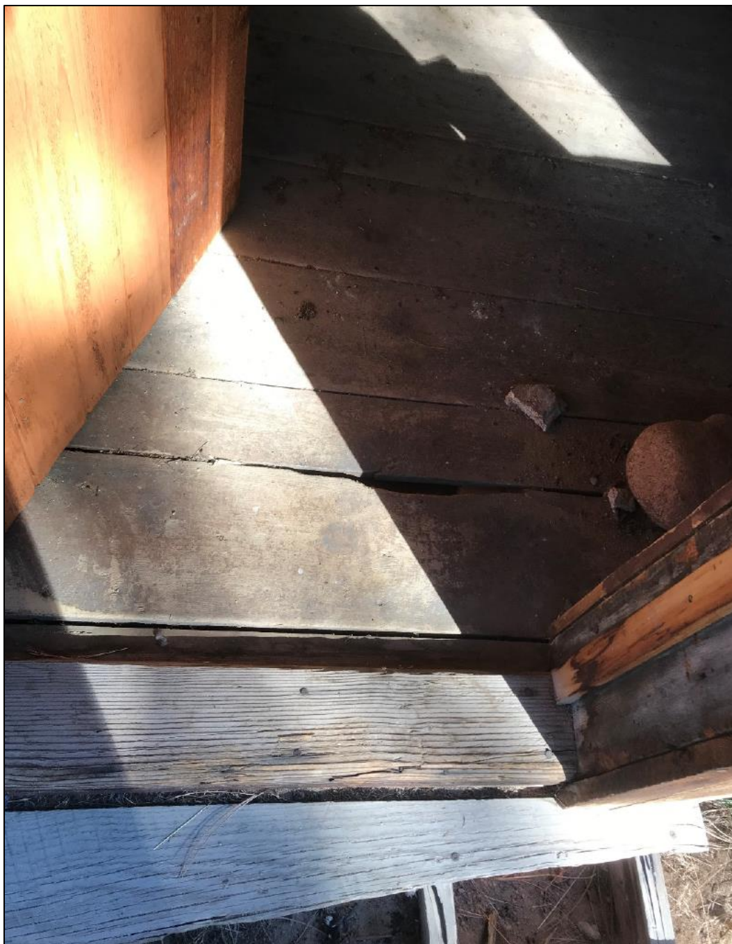
Figure 108. Floor planks inside the cabin's south door (photo by ERDC-CERL researchers, 2021).
