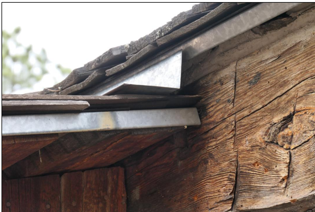
Figure 81. Galvanized metal edging along the porch roof planks on the east side of the Burgess-Capps Cabin (photo by ERDC-CERL researchers, 2021).
