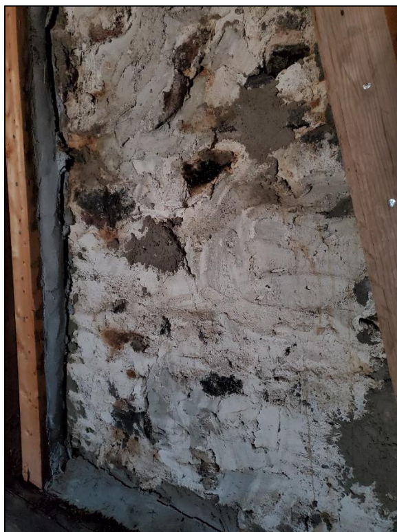
Figure 148. White mortar spread on the interior surface of the chimney (sample 17) (photo by ERDC-CERL researchers, 2021).
