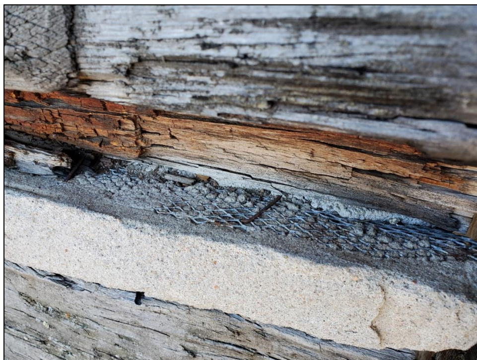
Figure 157. Example of nails and wire lath used as reinforcement for various layers of chinking (photo by ERDC-CERL researchers, 2021).
