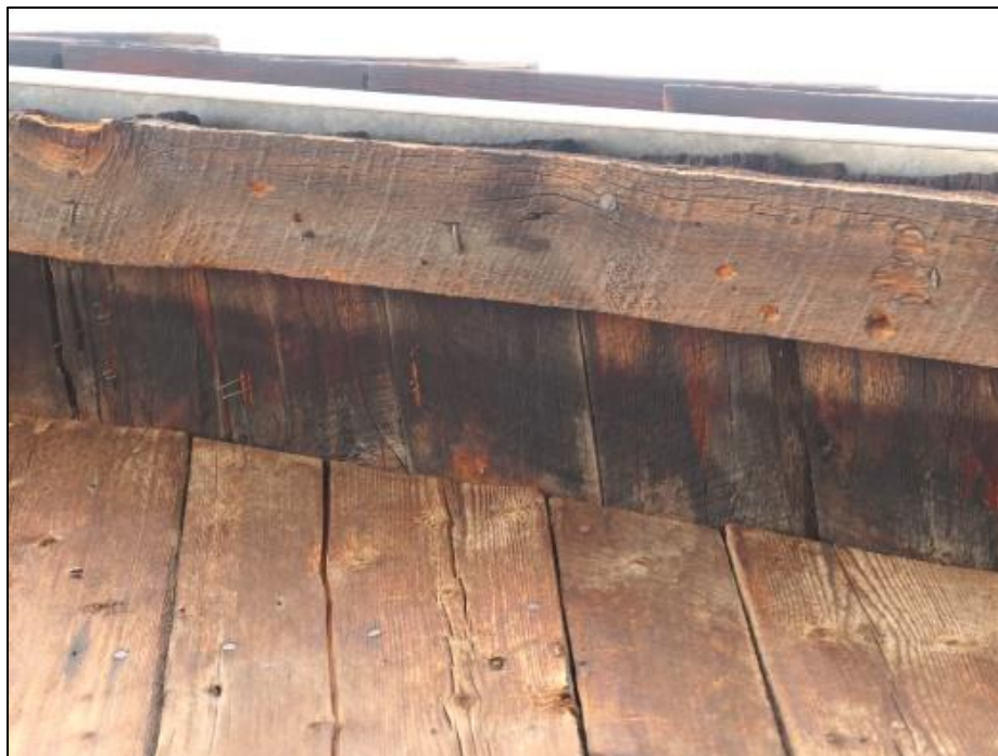
Figure 35. Looking at a closeup view of wood soffits and vertical siding along the gable of the Burgess-Capps Cabin (photo by ERDC-CERL researchers, 2021).
