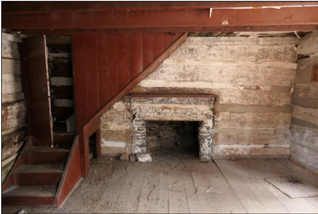
Figure 27. Looking at the fireplace and stairway on the east interior wall of the first floor of the Burgess-Capps Cabin (photo by ERDC-CERL researchers, 2021).
