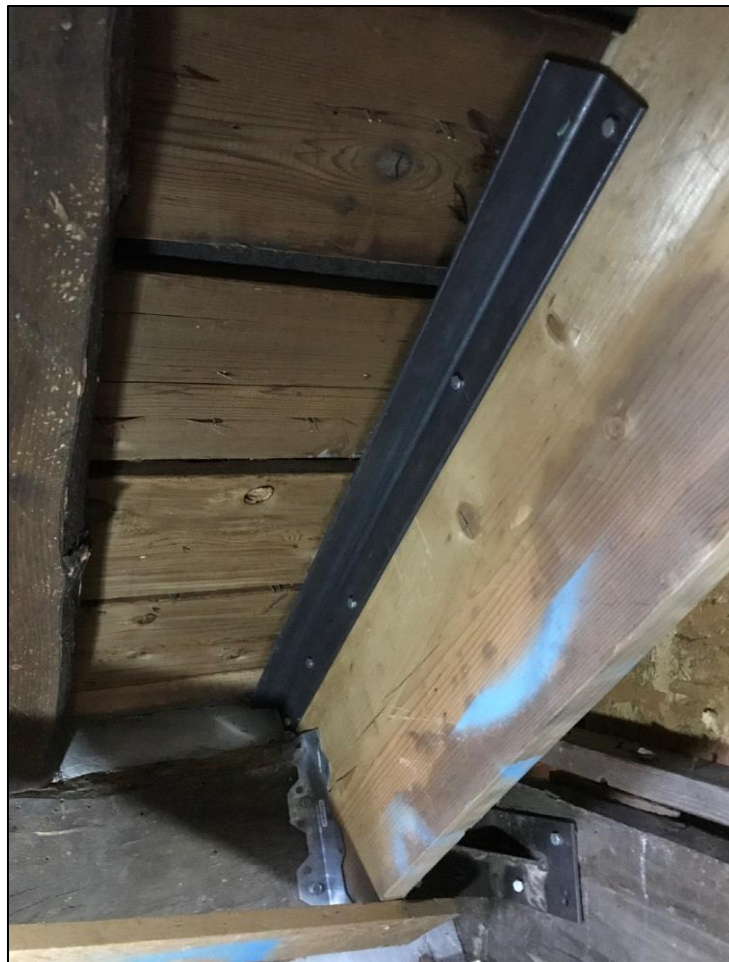
Figure 93. Bottom of 2 × 10 roof joists showing anchorage to top wall timbers using L2 × 2 × 1/8 in. angles in the Burgess-Capps Cabin (photo by ERDC-CERL researchers, 2021).
