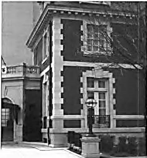
Figure 4. The foundation of this brick building is limestone, but the decorative trim above is architectural terra cotta intended to simulate stone.
