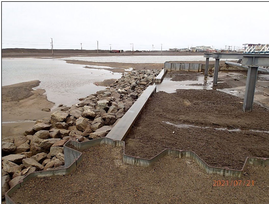
Figure 14. Itasigrook Dam spillway crest. (Image from CEPOA. Public domain.)
