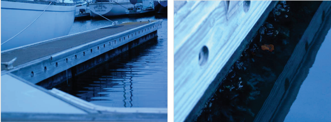
Figure 1. Example of marine hull fouling or biofouling. Sessile and mobile invertebrates grow on hard submerged surfaces such as docks and pilings ( left ). Close-up example of a hull-fouling community in San Francisco Bay, where the majority of the dominant species are aquatic nuisance species (ANS; right ). (Photo credit: S. Altman.)
