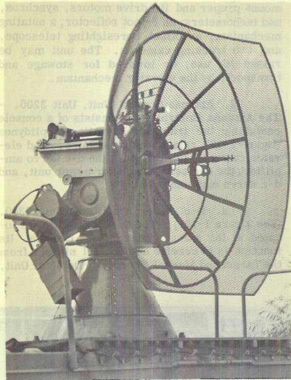
Figure 1-17. Antenna Unit - Front Oblique View
