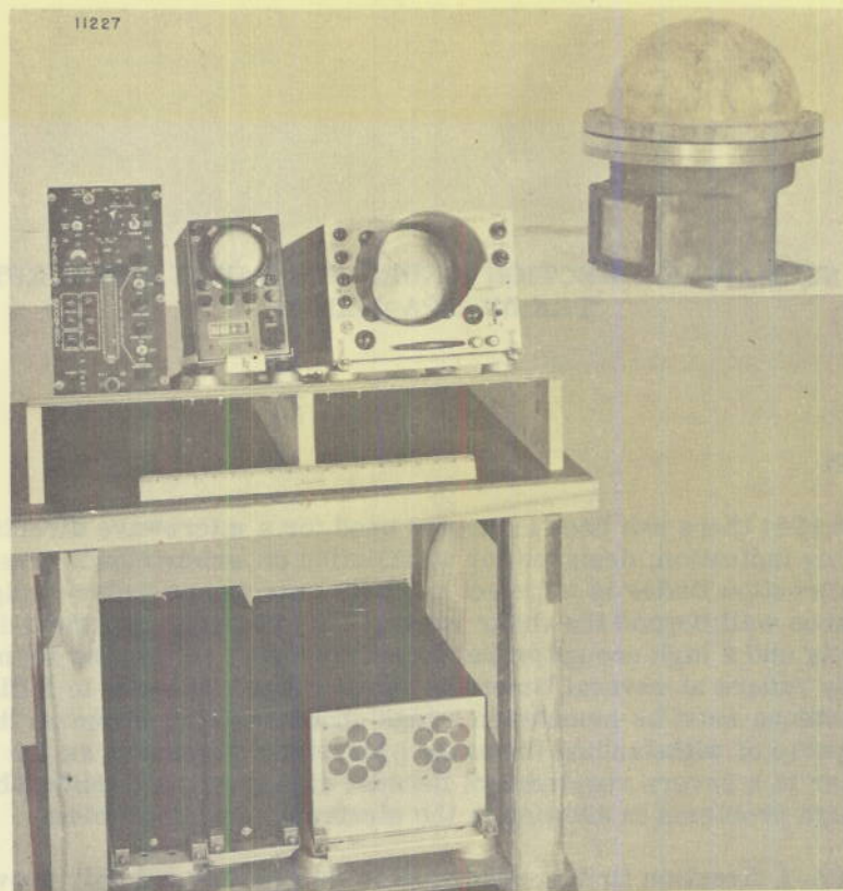
Figure 1 - Complete AN/BPA-1(XN-1) system
