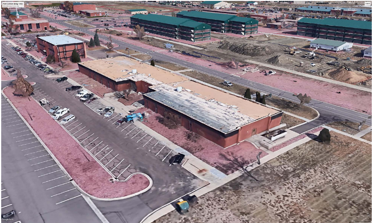
Figure 5.8. Fort Carson Office Building with Structure Elevation Relative to Ground
