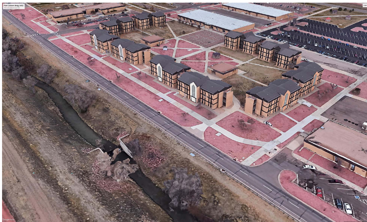
Figure 5.11. Fort Carson Barracks with an Estimate Class I Flood Hazard Source
