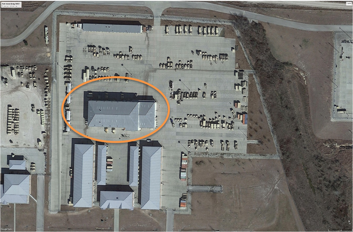
Figure 5.4. Vehicle Maintenance Shop at Fort Cavazos
