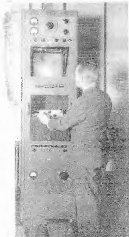
The electronically driven ripple tank showing a typical phase-front pattern in the viewing screen.
