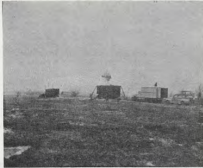
Figure 1 - SP-1M radar ground station
