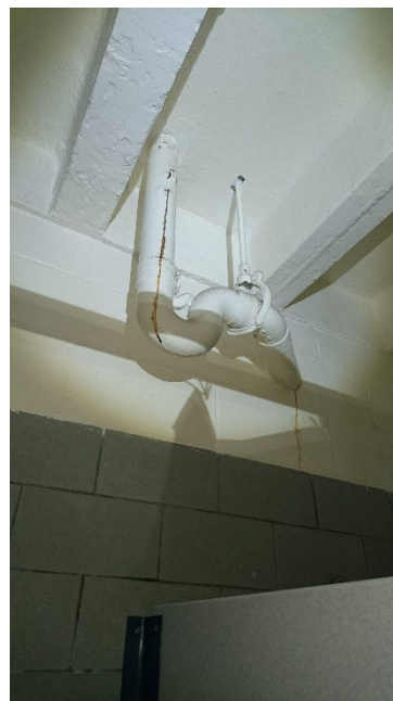
Figure 4.3. 3rd Floor Shower Drain and Drain Manifold. (Penetrated through floor to 2 nd floor ceiling)
