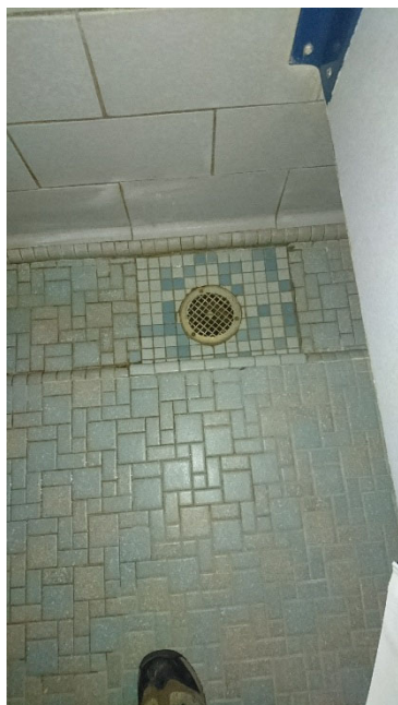
Figure 4.3. 3rd Floor Shower Drain and Drain Manifold. (Penetrated through floor to 2 nd floor ceiling)
