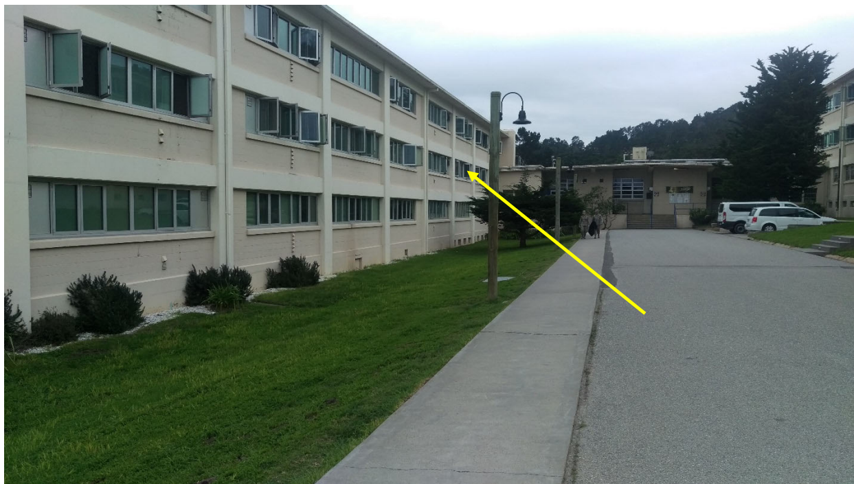
Figure 4.2. Building 627B Arrow points to showers location.
