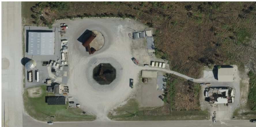
Figure 5. Aerial view of Silver Flag training site at Tyndall AFB
