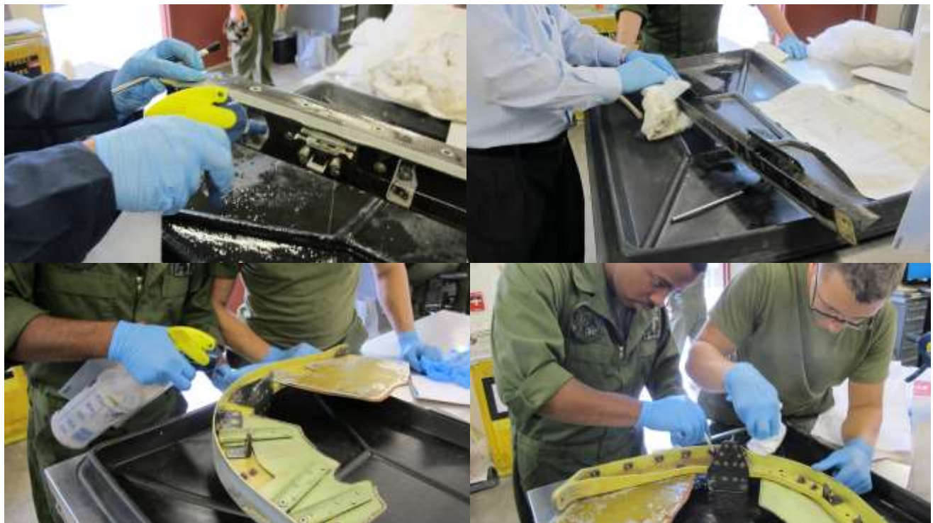
Figure 62. Cleaning trials on V-22 demonstration composite part
