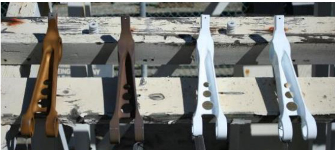
Figure 20. Corrosion Test Subjects on Installation (11/3/2014)
