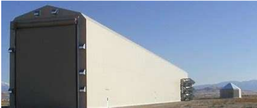
Looking down the long JABT from the west, inlet end.
