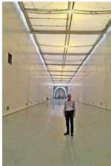
An inside view of the JABT.
