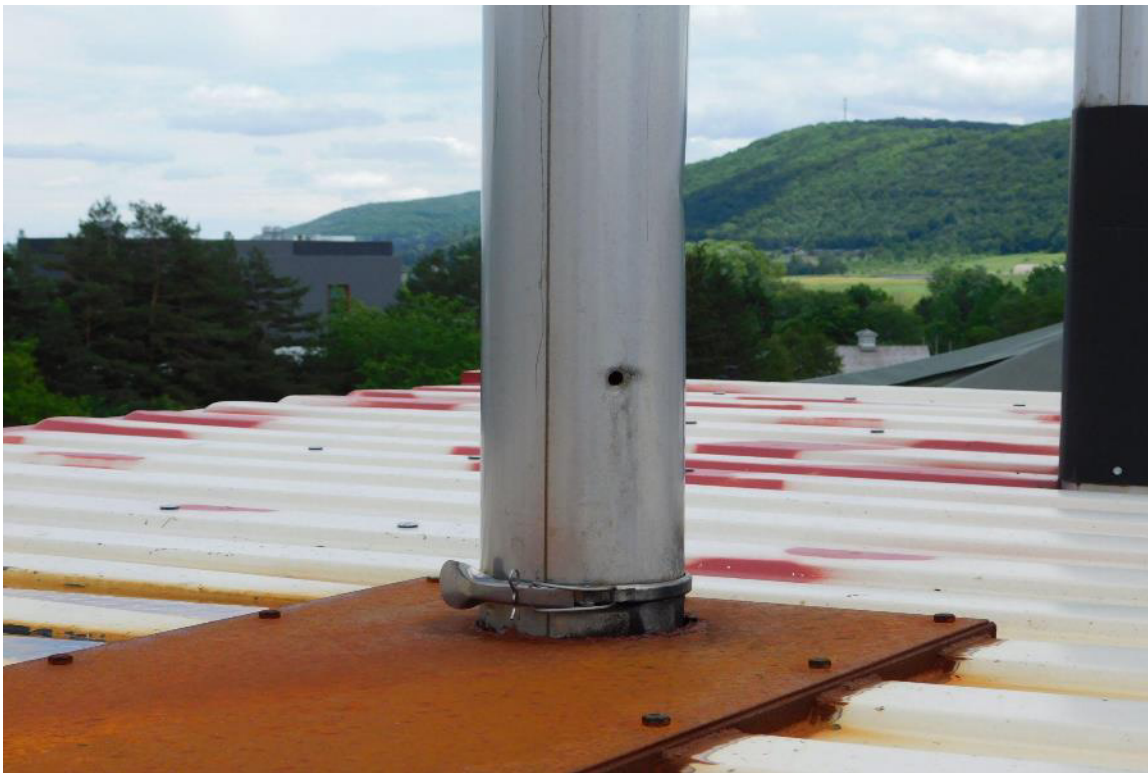
Figure 7.1. Combined Emissions Testing Port
