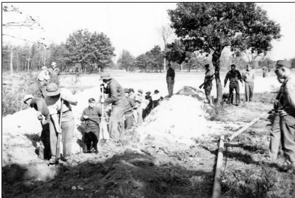
Figure 95. German POWs at Camp McCoy digging a trench, no date. (Image reproduced with permission from the David A. Yates Photograph Collection, Murphy Library Special Collections, University of Wisconsin–La Crosse.)
