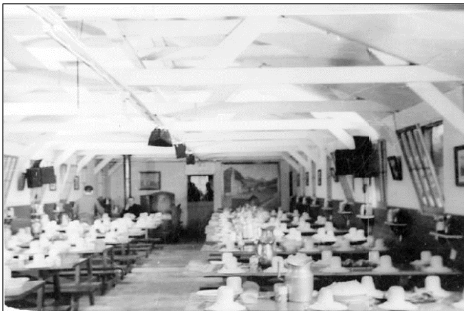
Figure 65. Interior of a German POW mess hall at Camp McCoy. (Image reproduced with permission from David Yates Collection, Murphy Library Special Collections.) 280
