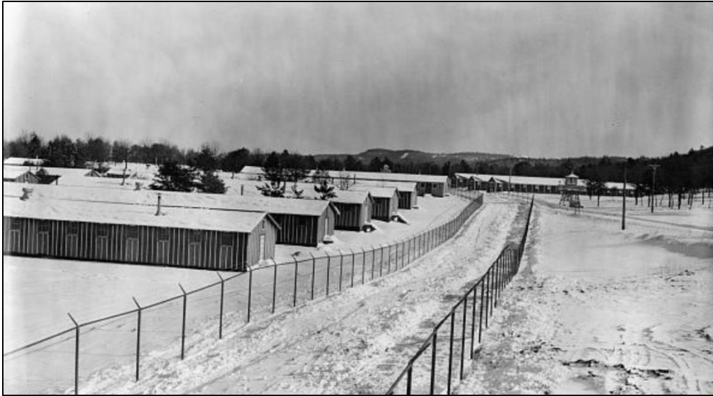
Figure 5. View of the parallel fence at the enemy alien compound, taken from guard tower 1601 in 1943. Looking southeast. (Image from Fort McCoy cultural resource manager [CRM]. Public domain.)
