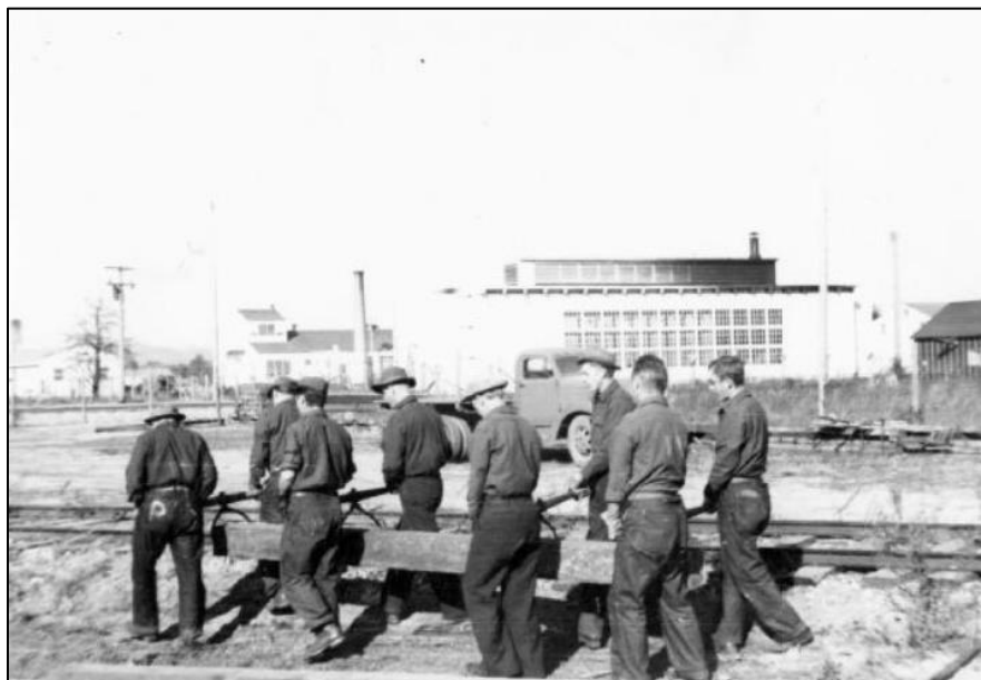
Figure 91. Eight German POWs repairing railroad ties at Camp McCoy, no date. (Image reproduced with permission from the David A. Yates Photograph Collection, Murphy Library Special Collections, University of Wisconsin–La Crosse.)
