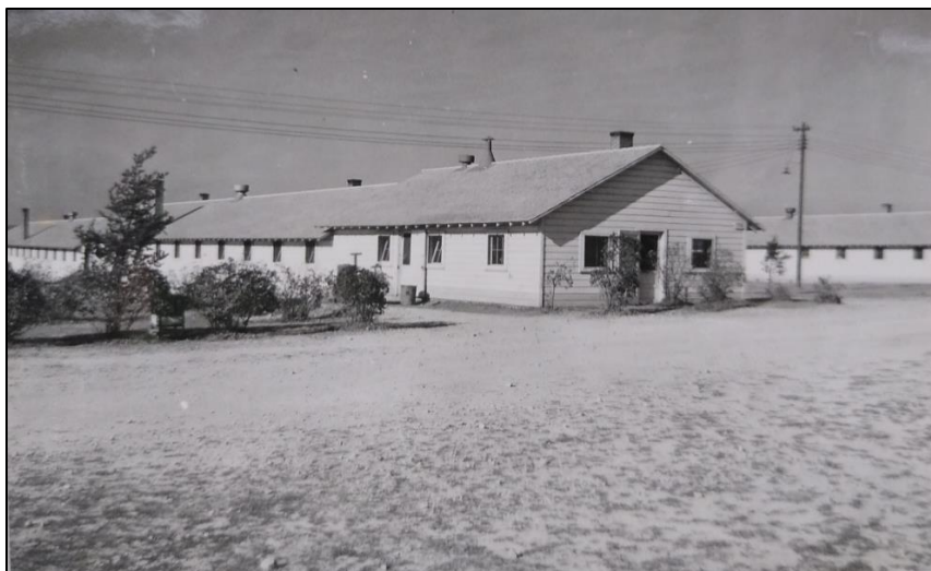
Figure 31. Exterior view of a Japanese barracks building in Compound C, 1944. (Image from NARA at College Park. Public domain.) 163
