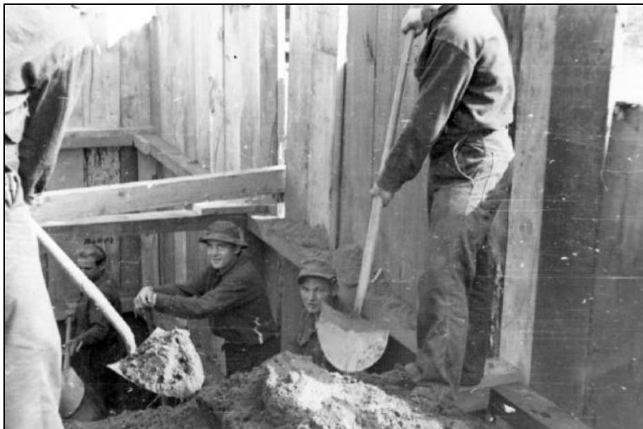
Figure 92. German POWs on an excavating detail, no date. (Image reproduced with permission from the David A. Yates Photograph Collection, Murphy Library Special Collections, University of Wisconsin–La Crosse.)
